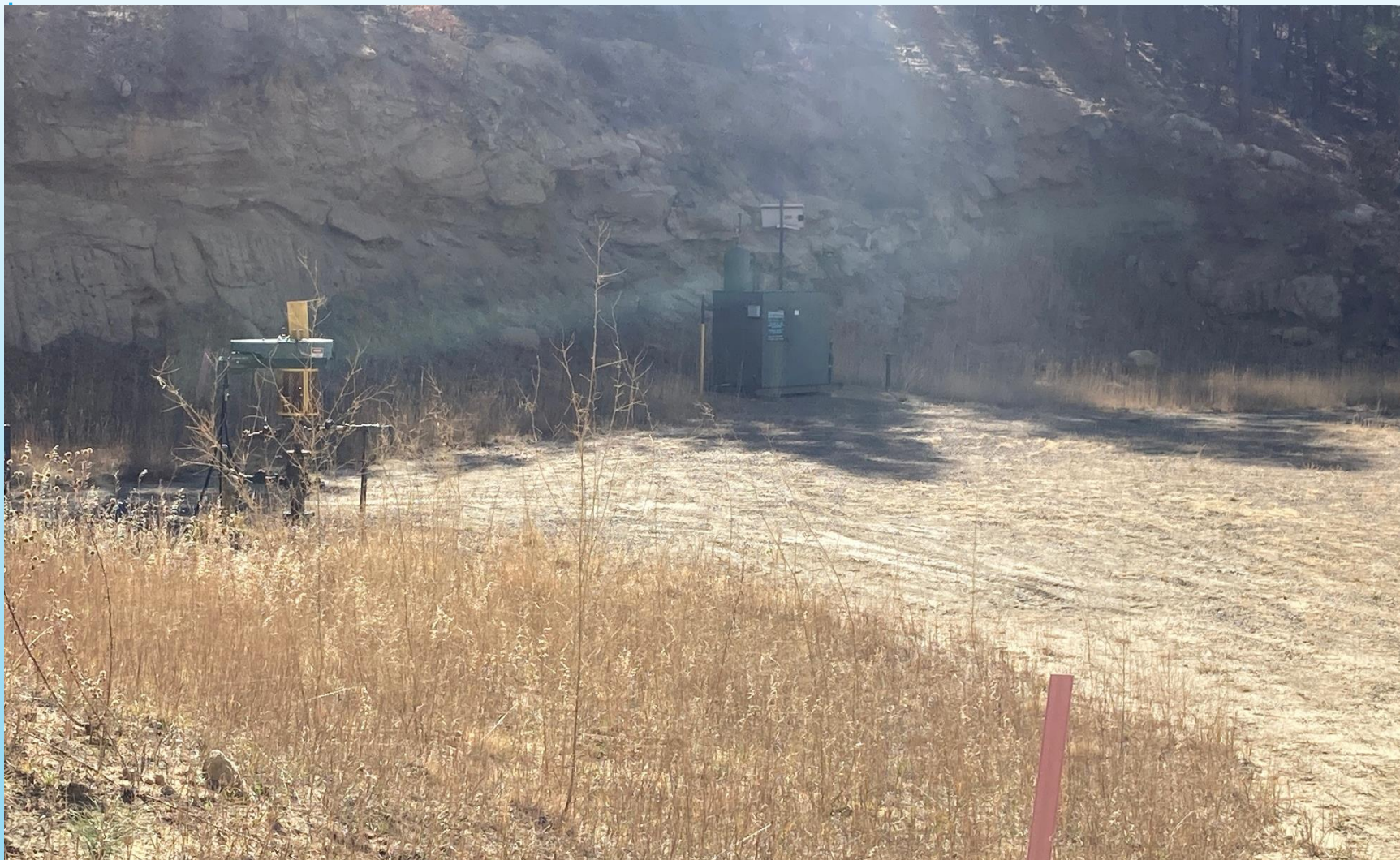
PHOTO 1: TR WELL PAD.
