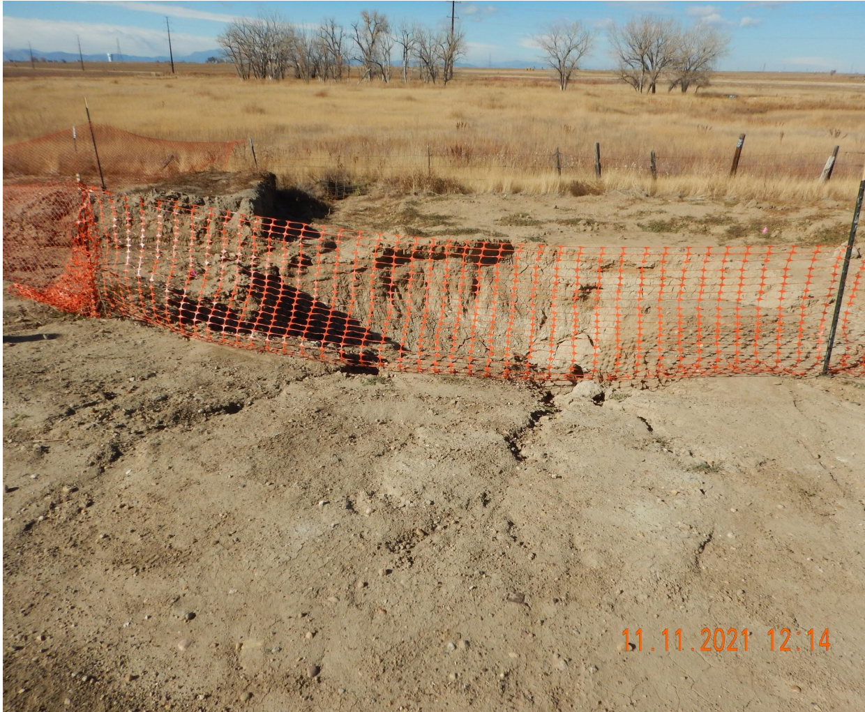
Photo 2. Photo taken from the remediation project, facing Northwest. Photo illustrates unmanaged run-on erosion into an open excavation with no outlet projection.
