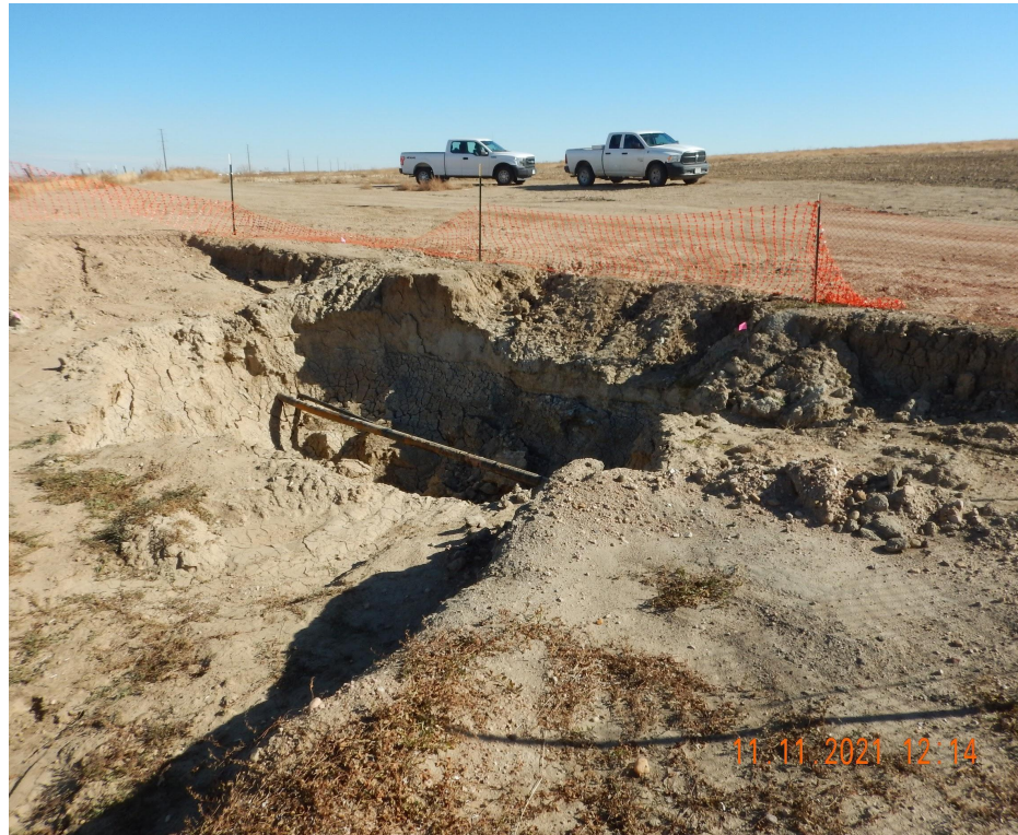
Photo 4. Photo taken from the remediation project, facing Southeast. See comments under Photo 2. Photo also illustrates an inadequate fence to prevent access when site is not attended.
