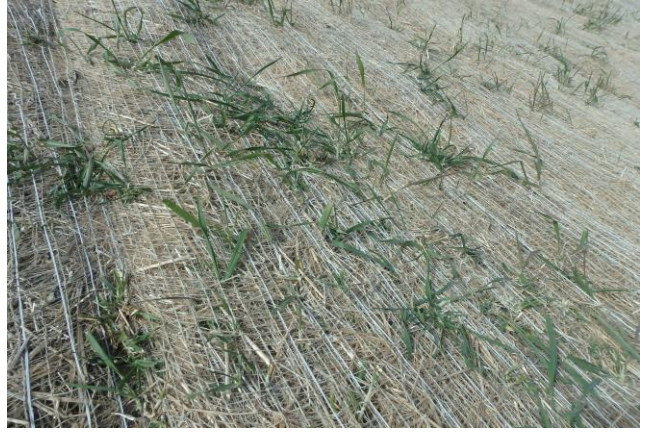
Temporary Seed Germinating through Erosion Control Blankets on the CC 697-09-61 Pad
