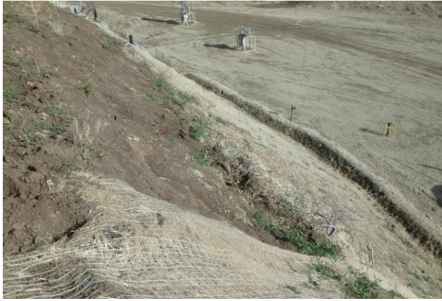
Steep Section of Cut Slope not Treated with Erosion Control Blankets on CC 697-09-61 Pad
