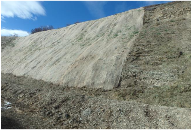
Damaged Erosion Control Blanket after Repairing on the Cascade Creek 697-09-61 Pad
