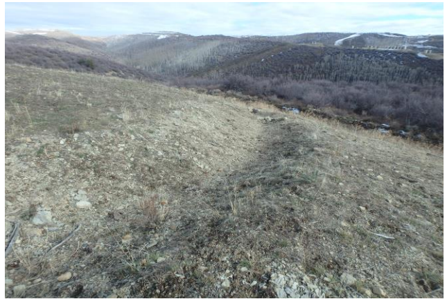
Outlet Channel on the CC 697-09-61 Pad Fill Slope
