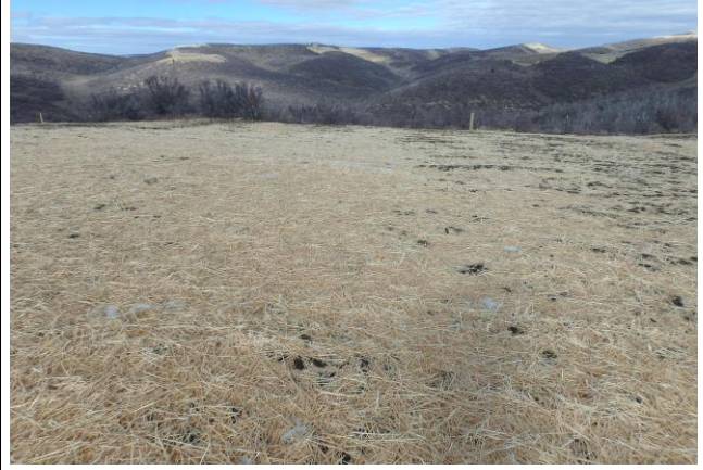
Straw Mulch Applied to the CC 697-08-53 Pad
