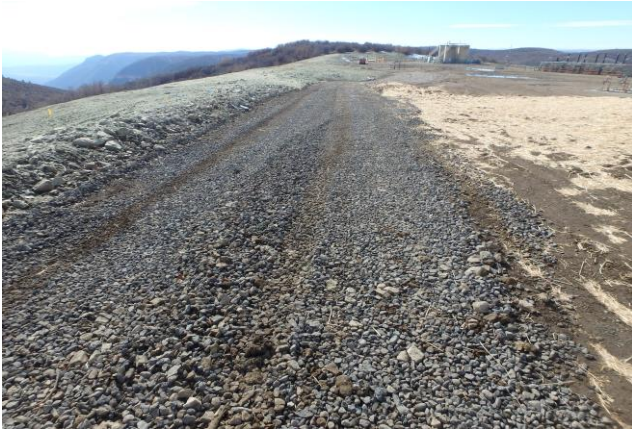
Clean Gravel Applied to the CC 697-08-53 Access Road
