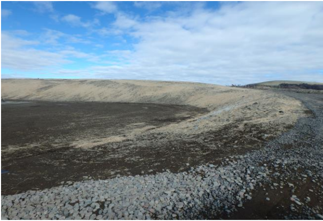
Straw Mulch Applied to the CC 697-08-53 Pad
