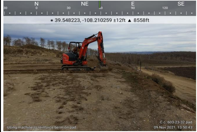
Installing Earthen Berm on the Cascade Creek 603-23-32 Pad
