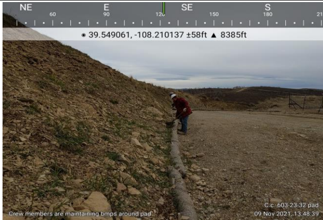
Maintaining Existing Wattle Installations on the Cascade Creek 603-23-32 Pad
