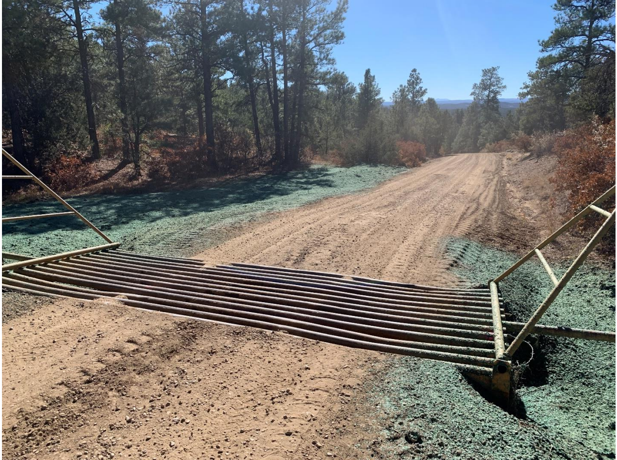
Cattleguard was cleaned of sediment and reseeded
