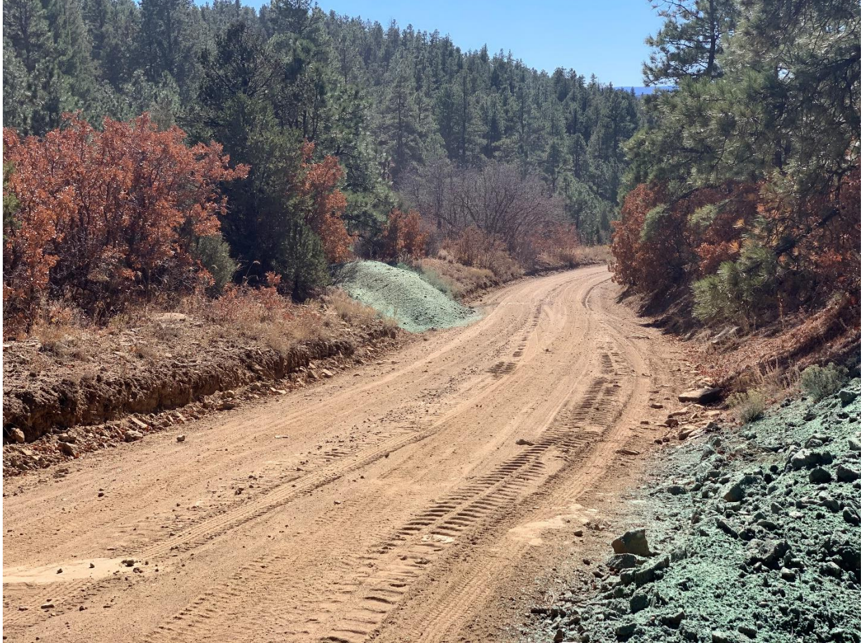
Repaired areas of vehicle tracks and rutting to comply with rule 1002.e. Reseeded disturbed areas Installed or repaired required BMPs per Rule 1002.f.(2)C
