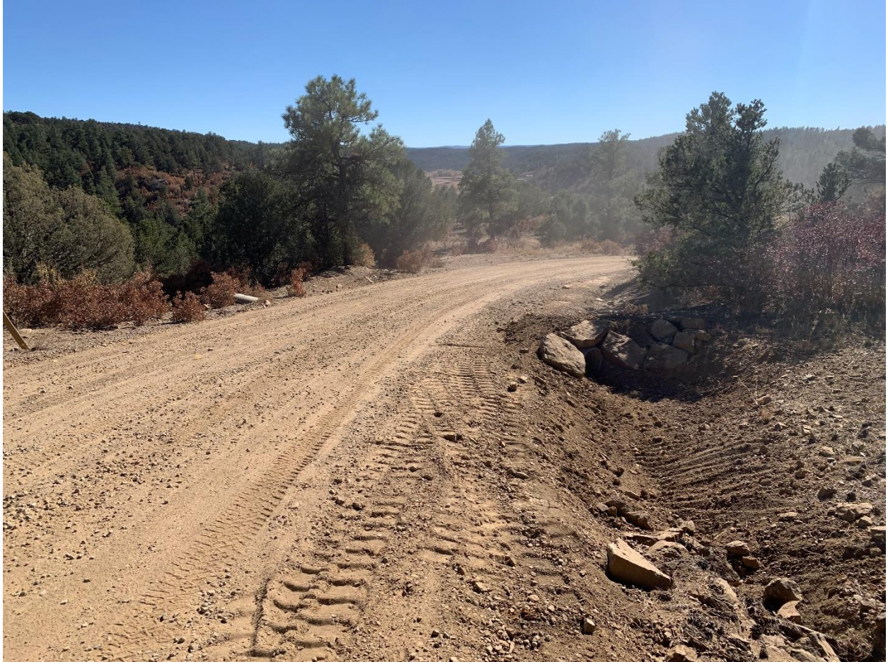
Repaired areas of vehicle tracks and rutting to comply with rule 1002.e.
