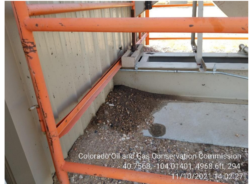
Photo 4 – Stained Soil at Gas Engine
