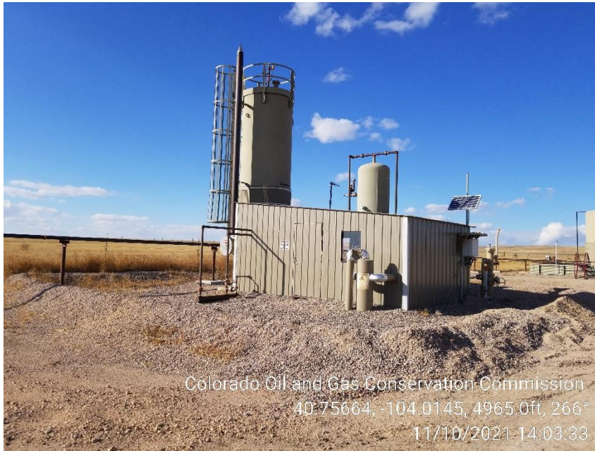
Photo 7 – Heater Treater
