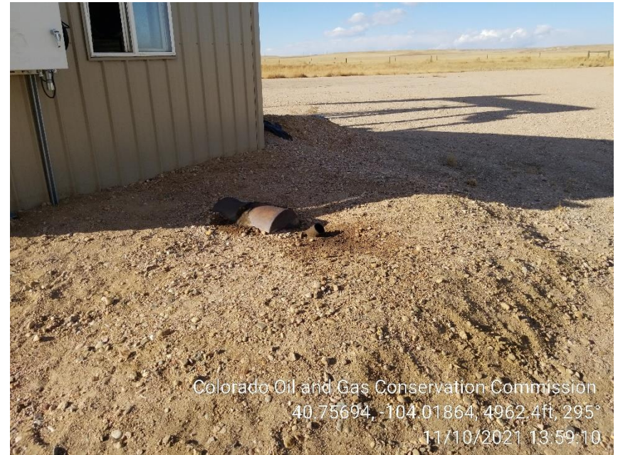
Photo 6 – Stained Soil at Exhaust
