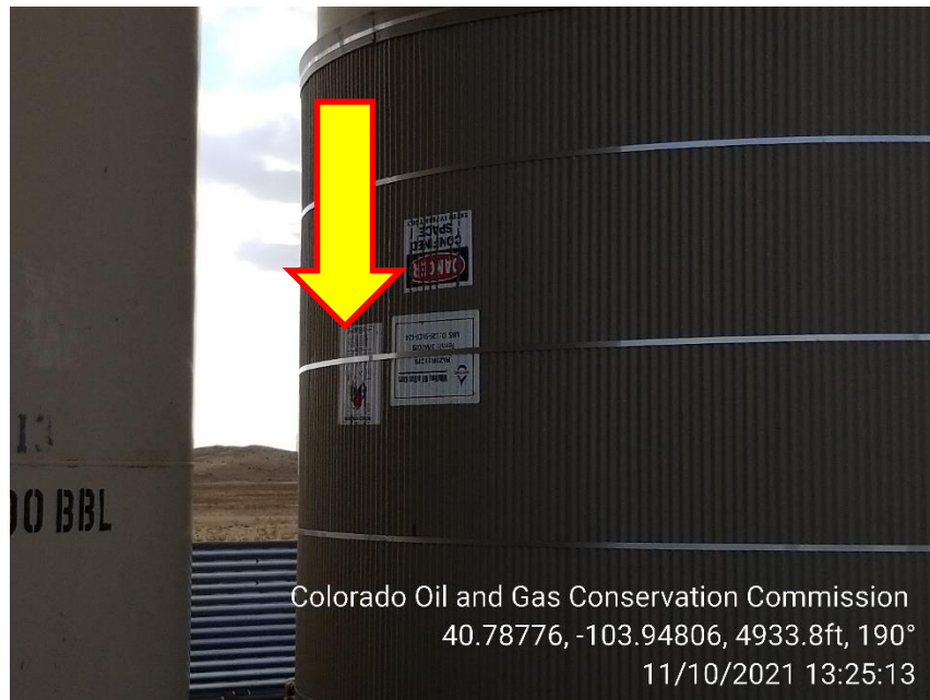
Photo 3 – Labels Upside down and not visible
