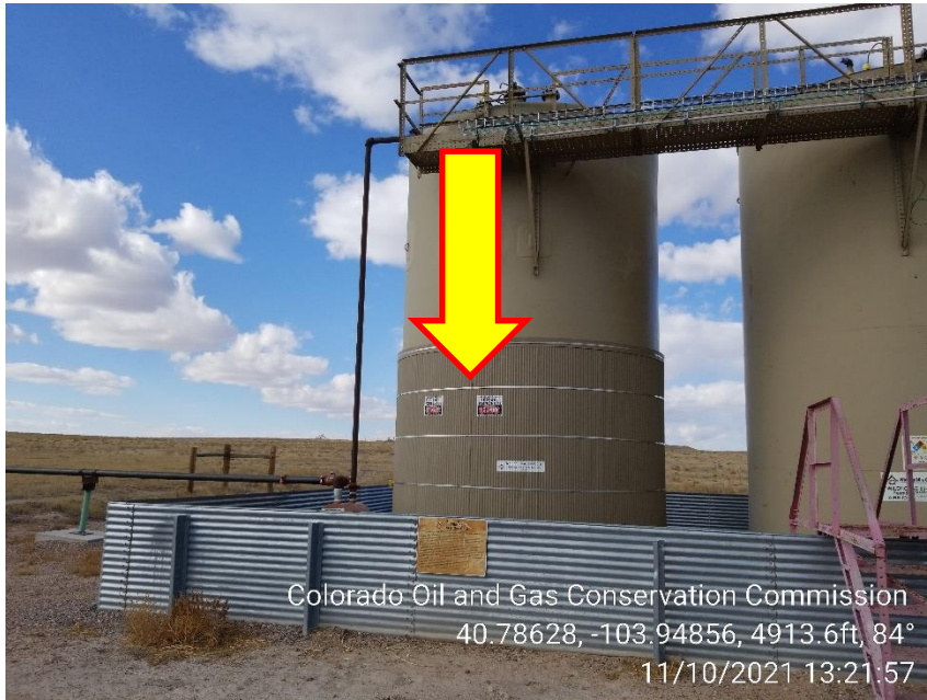
Photo 9 – Produced Water Tank missing NFPA, Content and Capacity
