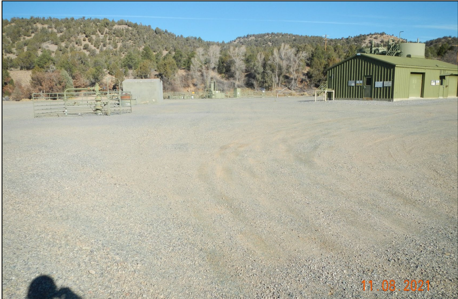
Photo 1. View of the project area from the well pad entrance facing center. Debris observed during previous inspection is not observed.
