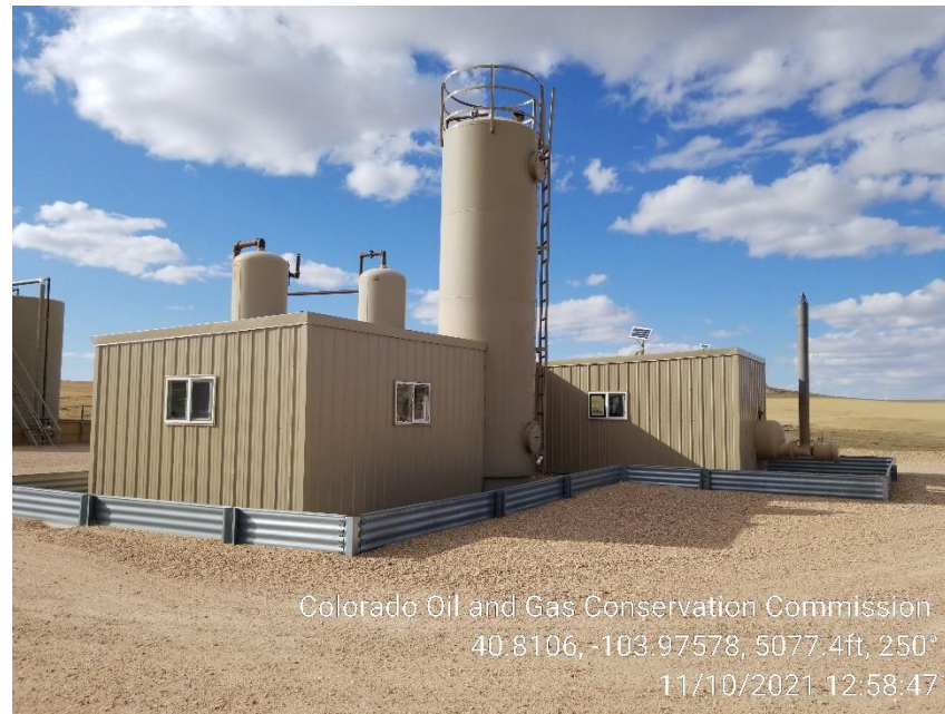
Photo 2 – East Heater Treater
