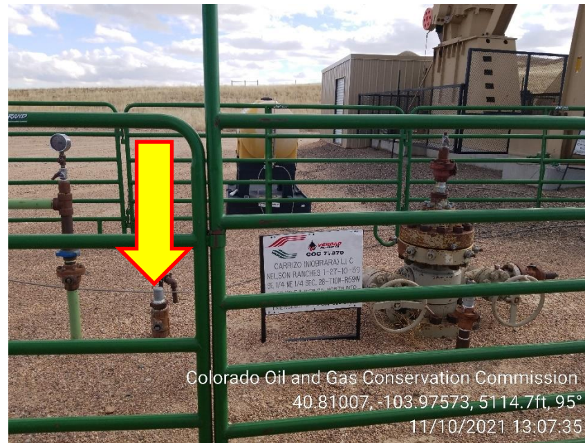
Photo 8 – Unmarked Riser at 1-27-10-59 Wellhead
