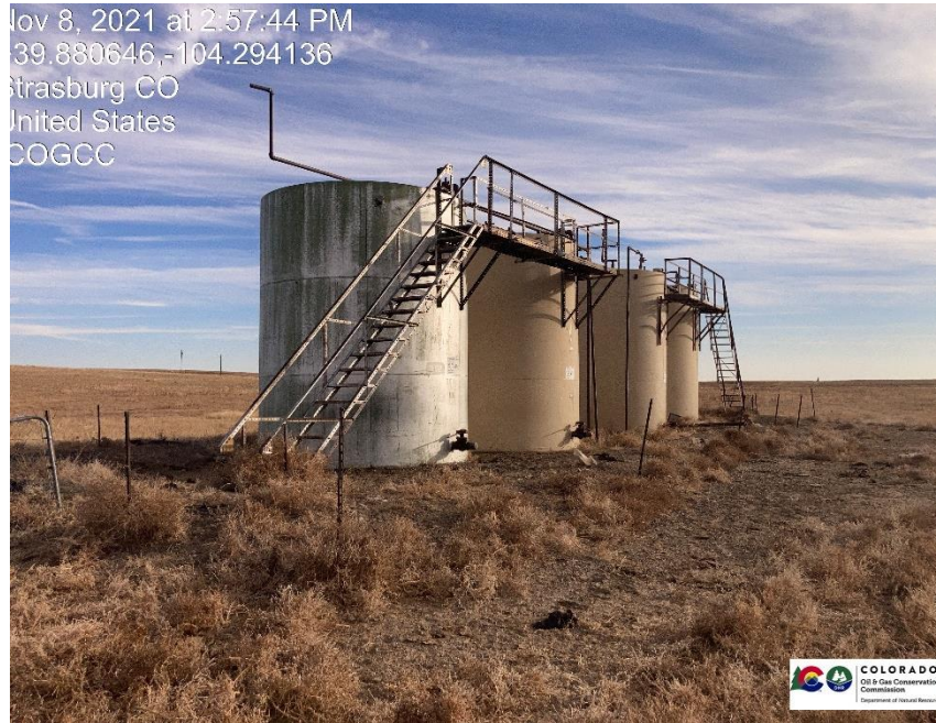
Pic 3 Tank battery, weeds unmanaged on location, fence needs to be repaired, Berm needs to be repaired.
