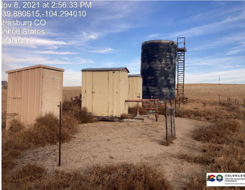
Pic 5 gas meter run on location, unable to inspect calibration due to weed growth on location, weeds unmanaged.
