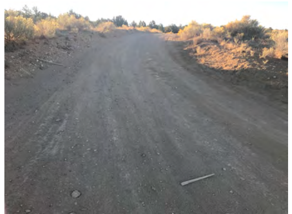
PAD ACCESS LOOKING EASTERLY
