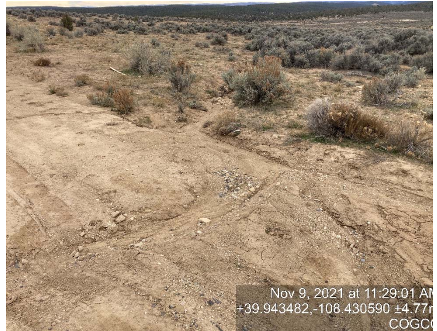
Lack of stabilization/erosion/sediment migration
