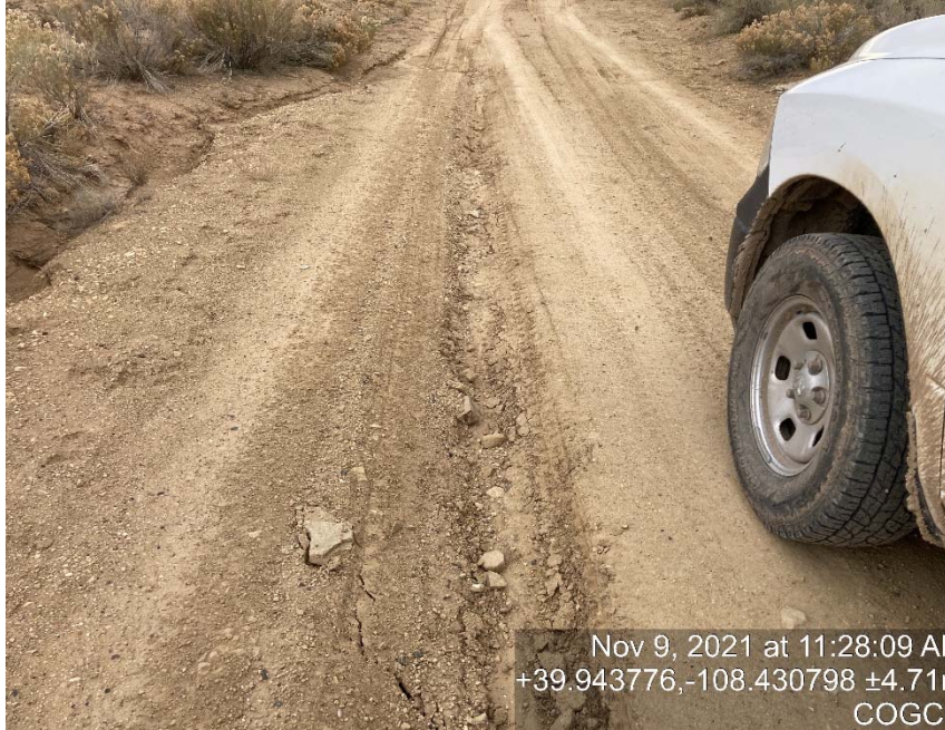
Lack of stabilization/erosion
