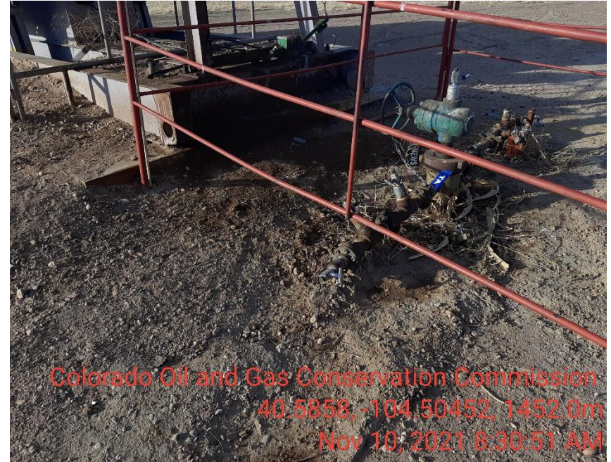
Photo 2 Stained soil around well head
