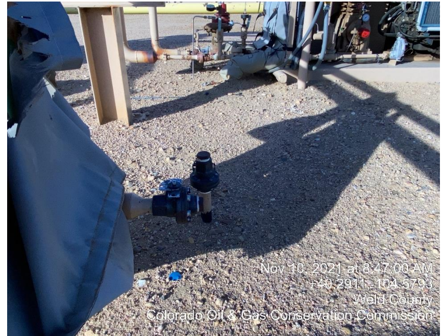
Photo #4 Unmarked riser
