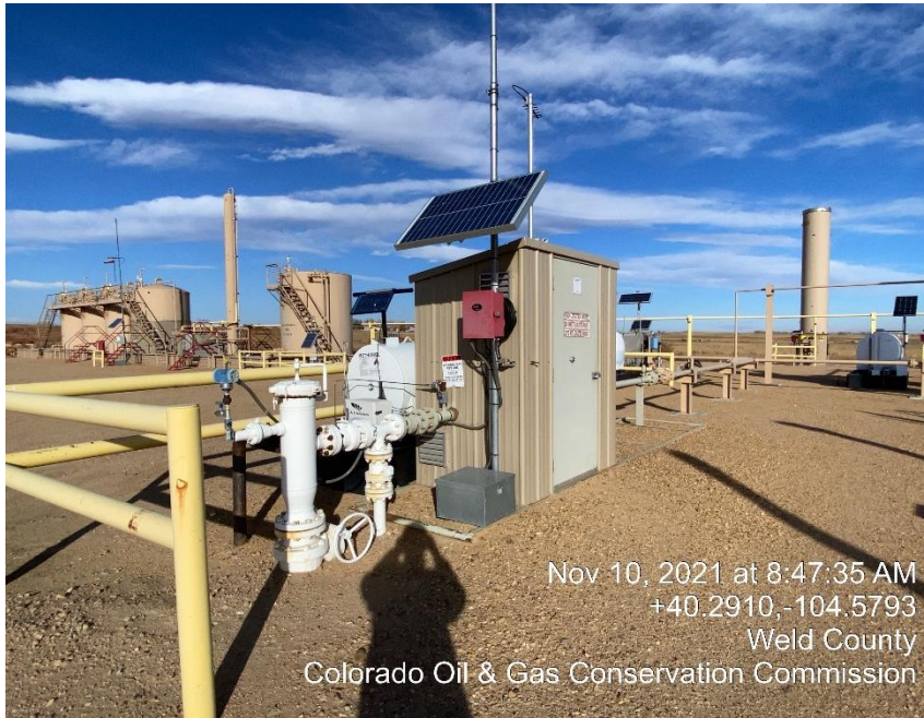
Photo #3 Gas Meter Run
