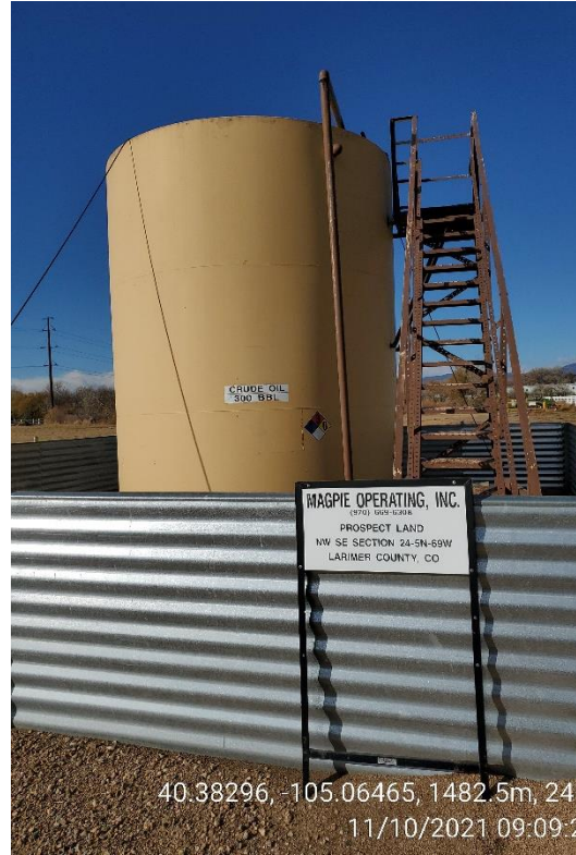
Photo 2 Crude Oil Tank
