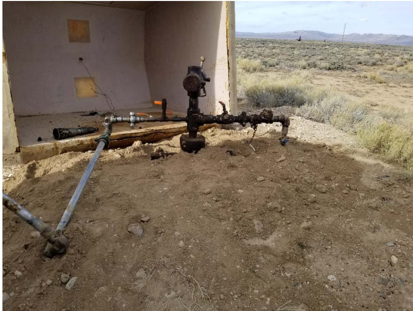
Photo 1. No bradenhead access apparent.
