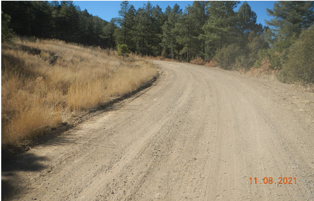
Photo 1. Facing southwest along the access road. The road has been regraded.
