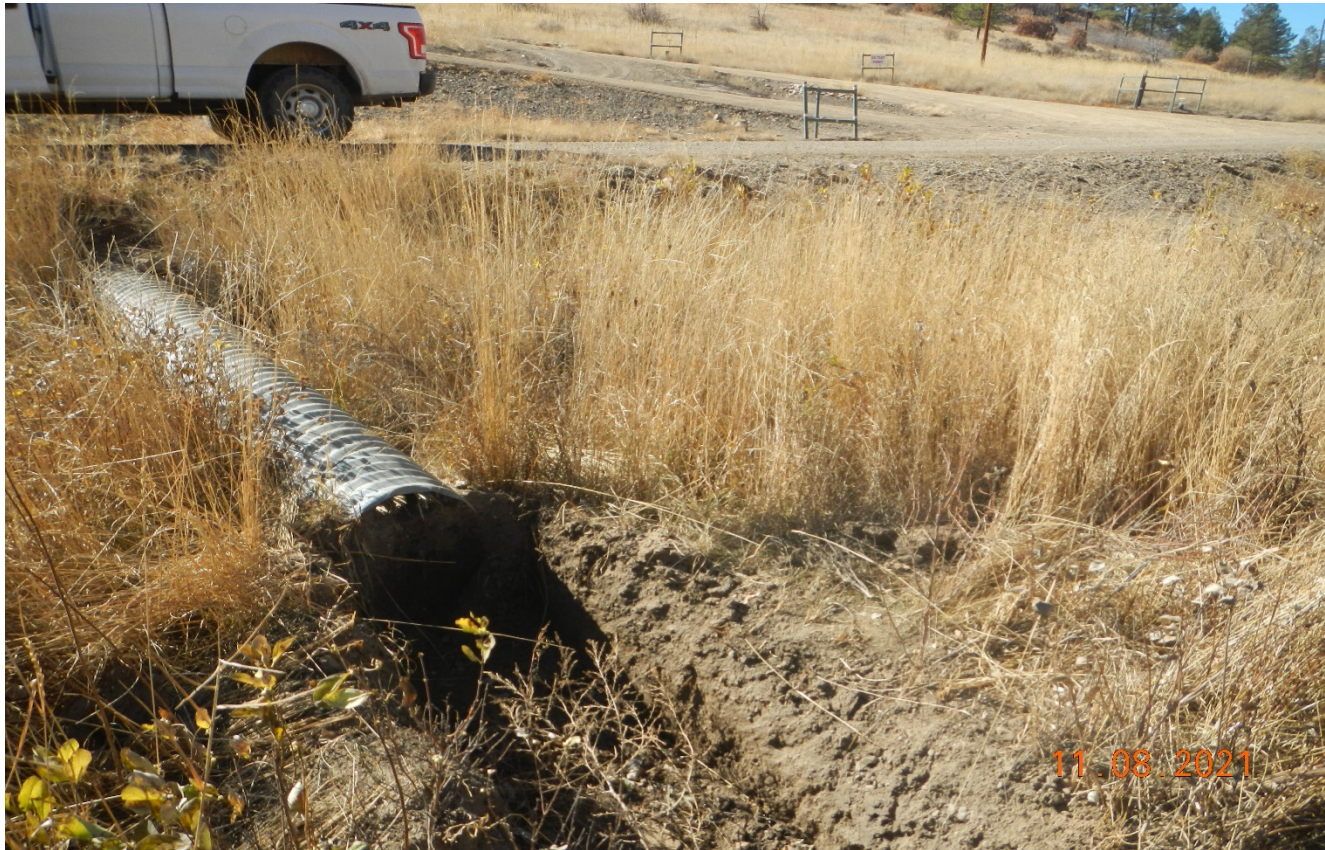
Photo 3. The culvert near the location on the main road is still filled in with sediment.
