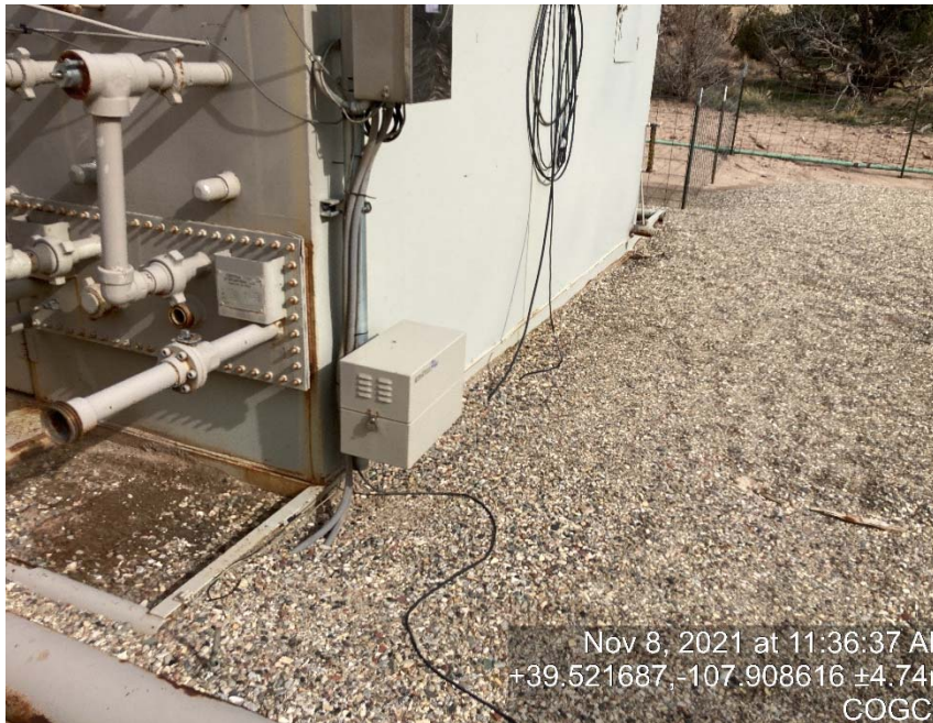
Glycol vessel missing labeling
