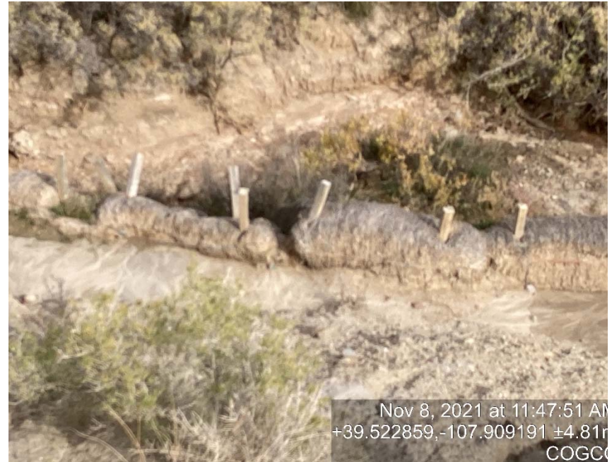
BMP'S failing off edge of location on N/E side of wells
