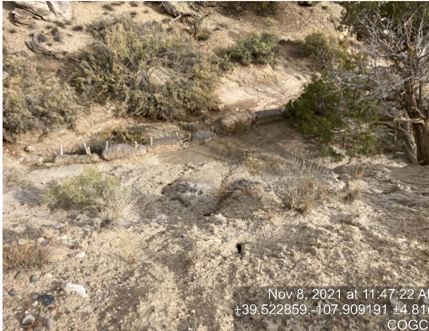
BMP'S failing off edge of location on N/E side of wells
