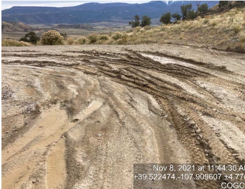
Lack of stabilization/ compaction
