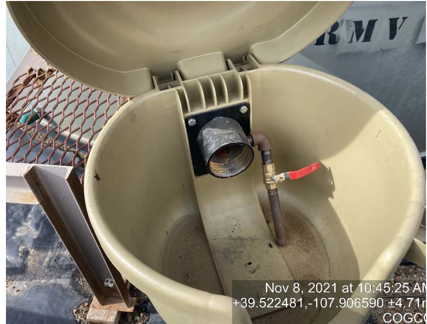
Load lines missing caps/bull plugs
