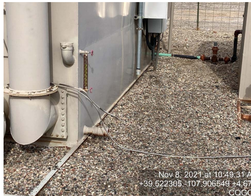
Glycol vessel missing labeling
