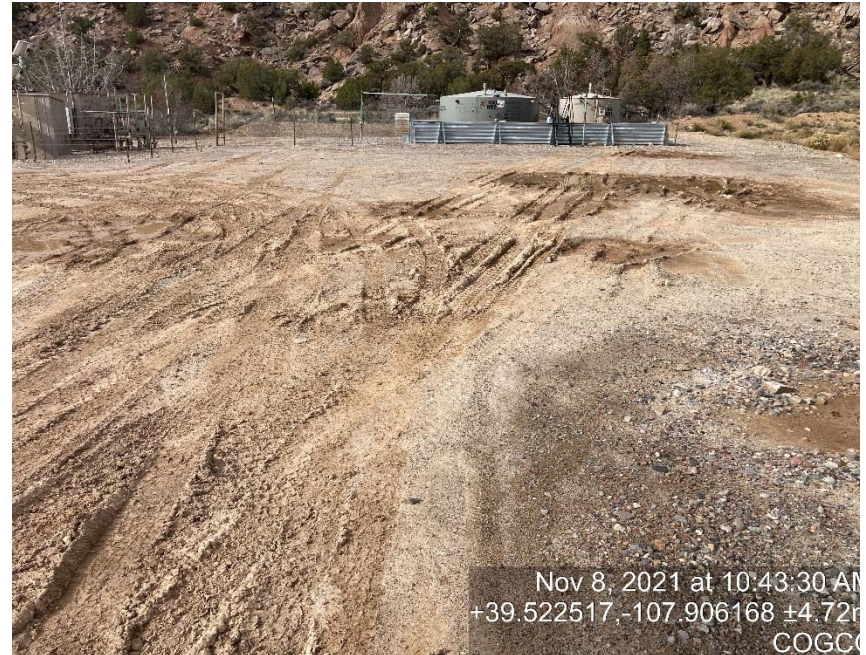
Lack of stabilization/compaction
