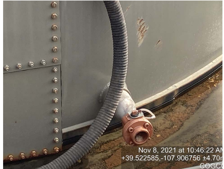
Load lines missing caps/bull plugs
