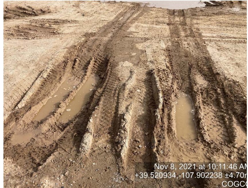
Follow up inspection of lack of stabilization/ compaction
