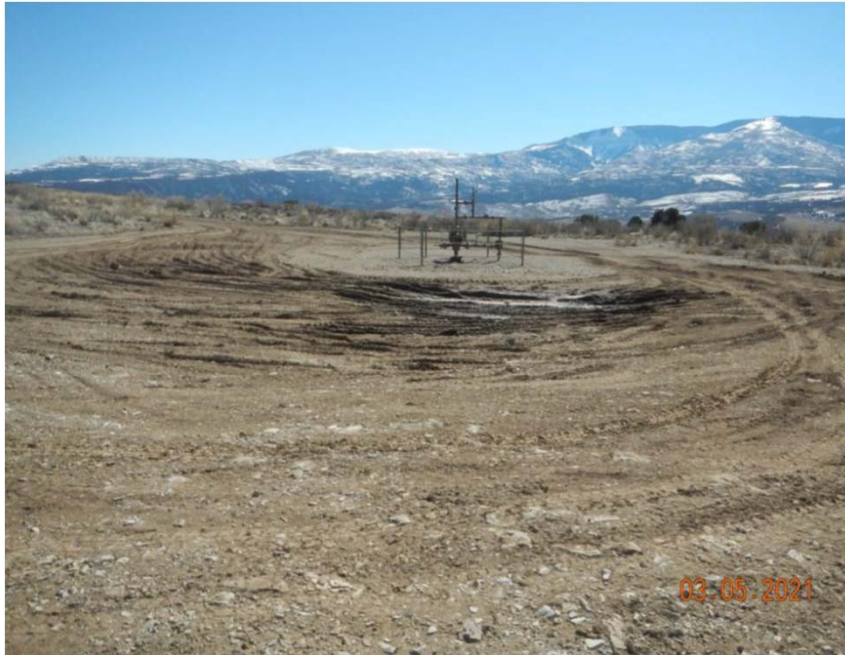
Previous inspection of lack of stabilization/ compaction
