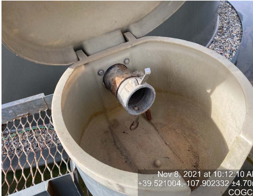
Load out lines missing caps/bull plugs
