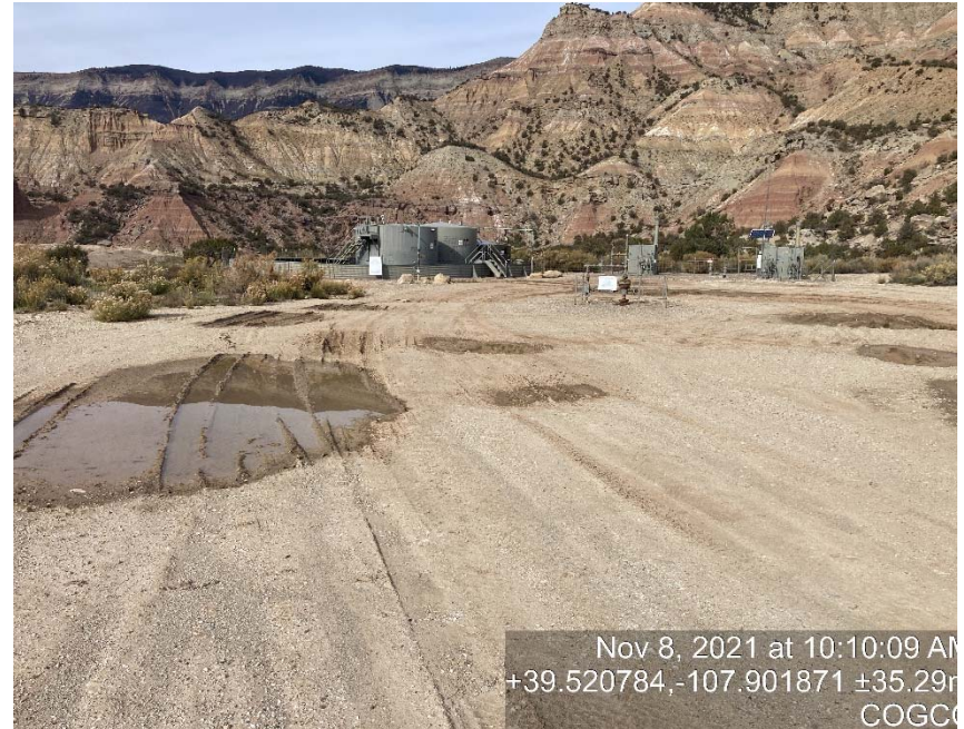
location/Lack of stabilization/compaction
