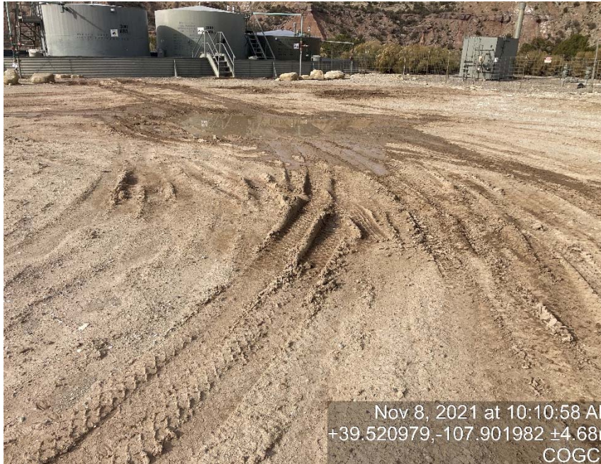
Lack of stabilization/compaction
