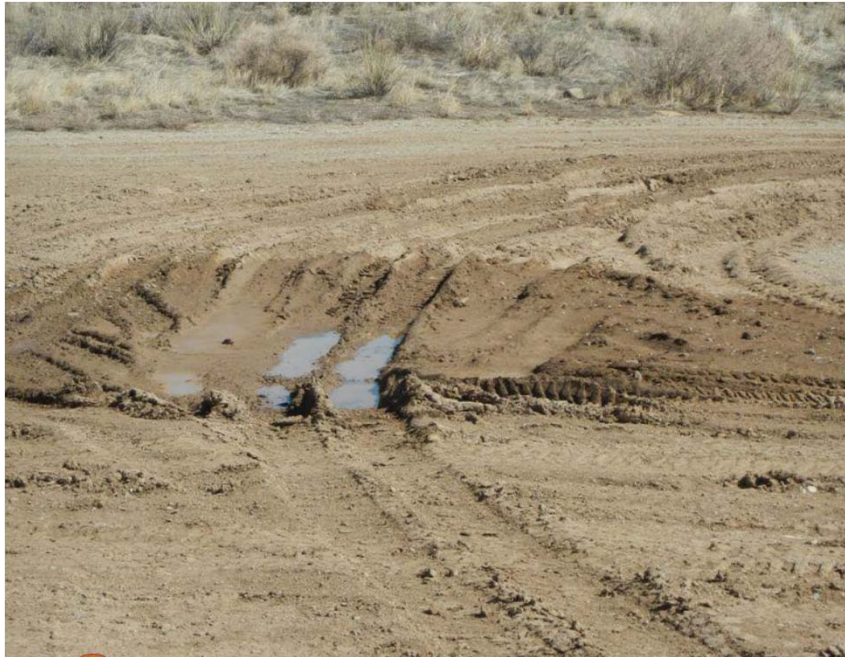
Previous inspection of lack of stabilization/ compaction
