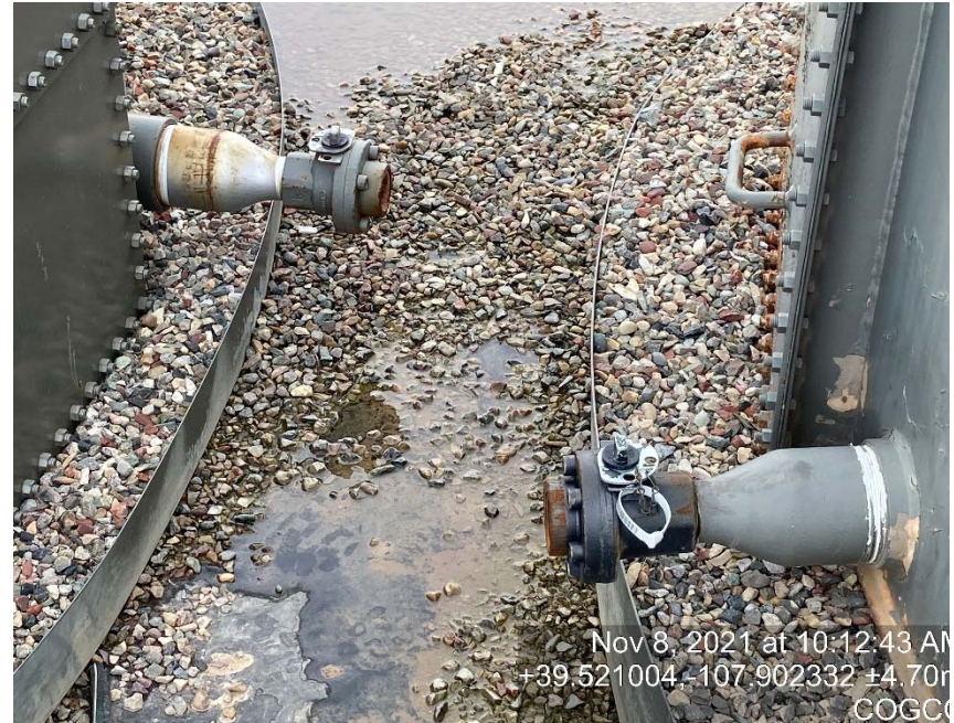
Load out lines missing caps/bull plugs
