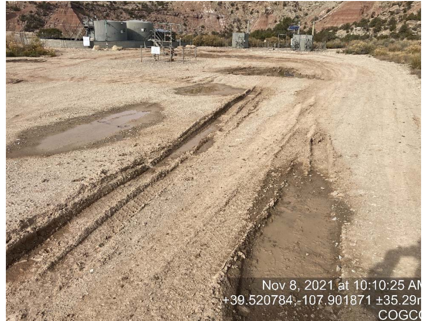
Lack of stabilization/compaction
