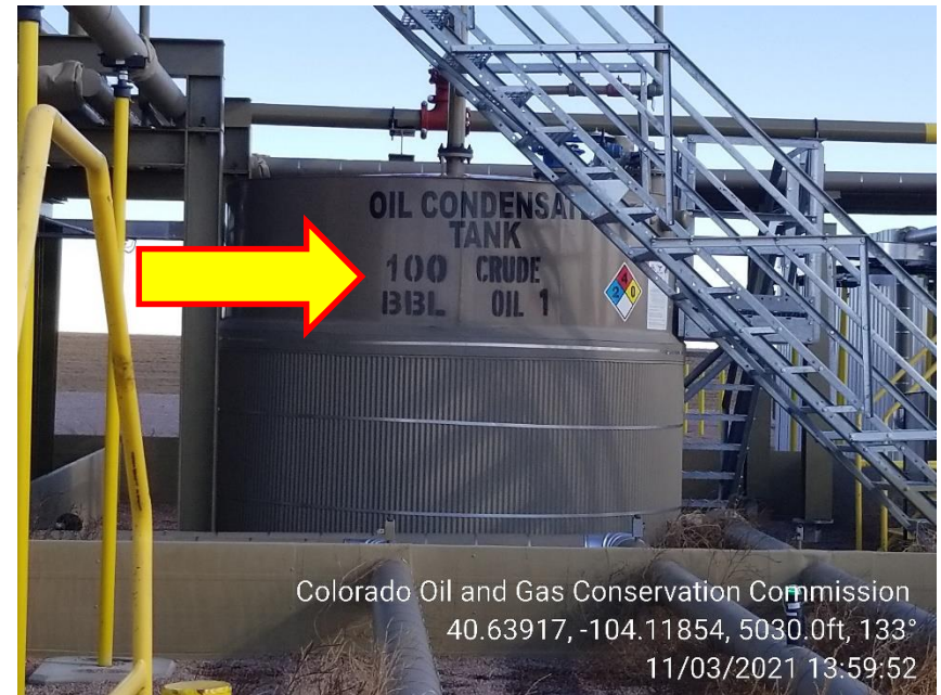
Photo 2 – Capacity Label installed
