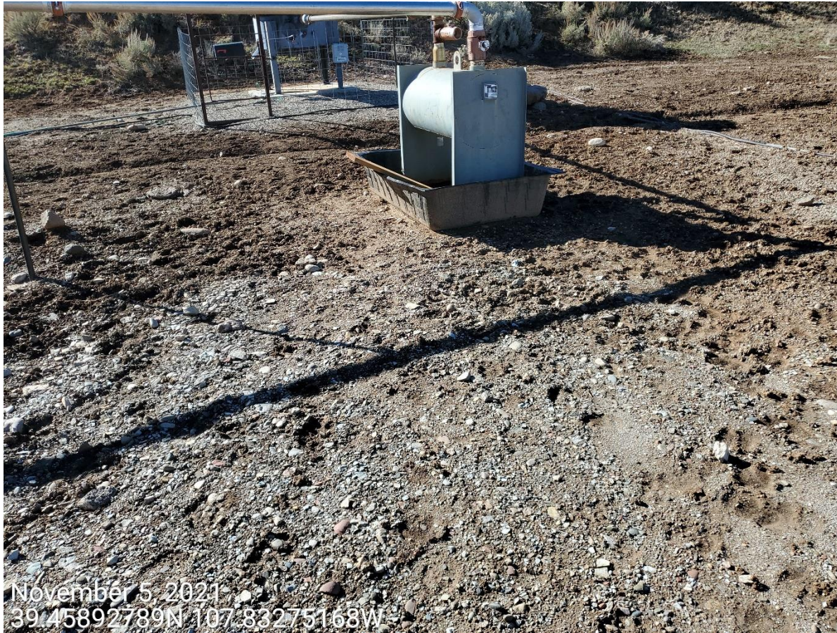
Photo 1: Photo shows wildlife protection devices to prevent wildlife access to the containment BMP remains missing or insufficient.
