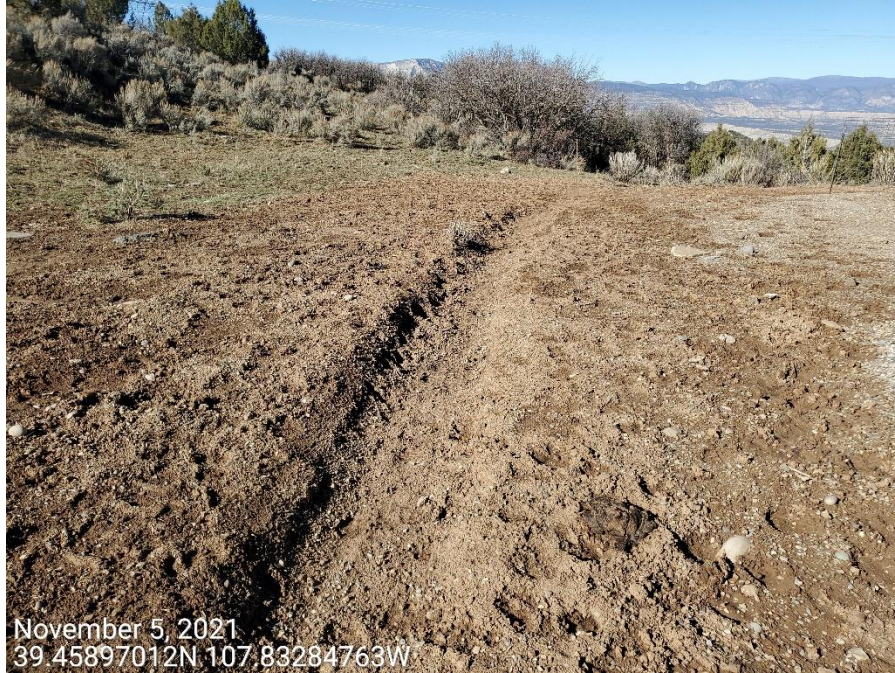
Photo 2: Photo taken from the stormwater diversion ditch on the west end of the Location, facing north. Photo shows that the stormwater diversion ditch remains improperly constructed with an outlet, to prevent offsite degradation due to runoff.
