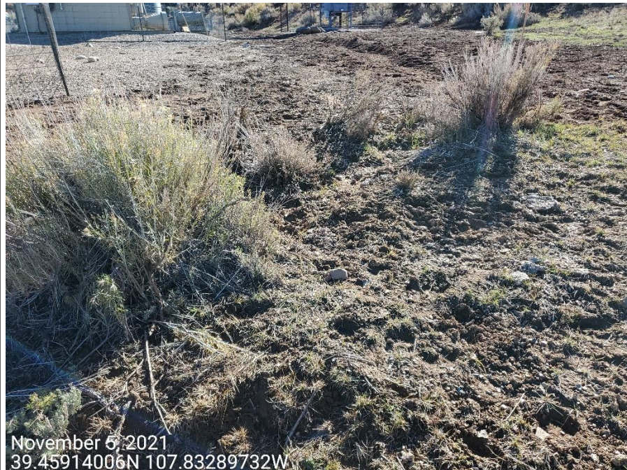
Photo 3: Photos taken north of the ditch. Photo shows offsite erosion degradation due to improper stormwater runoff controls on the Location.
