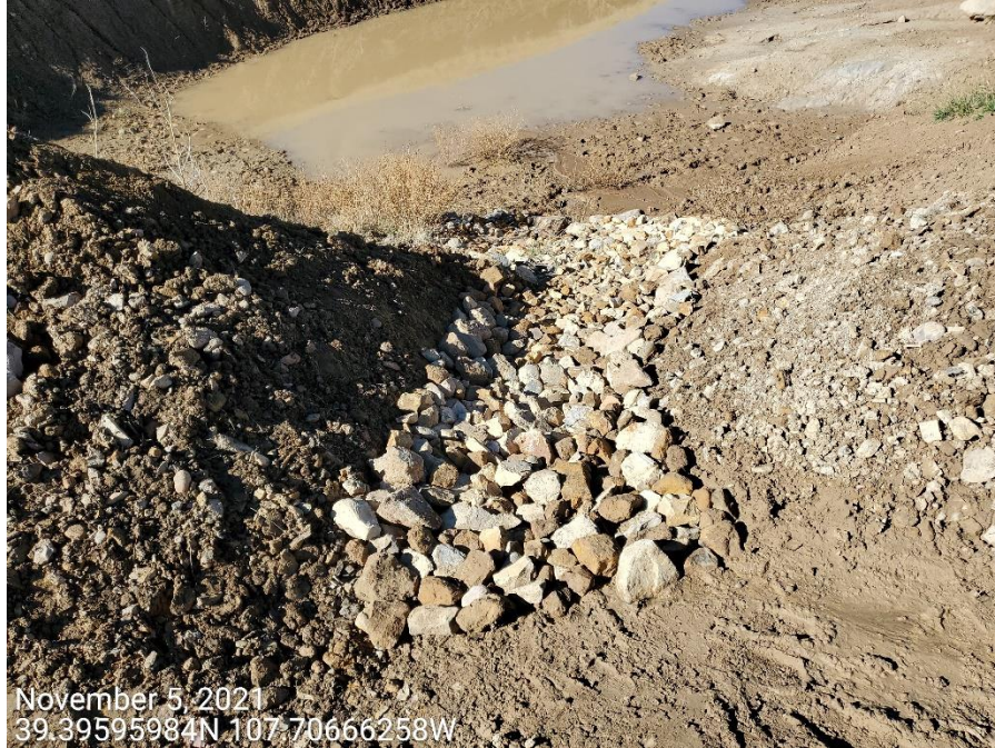
Photo 4: Photos shows the outlet from the production area leading into the sediment trap is improperly armored and missing geotextile lining per good engineering practices.
