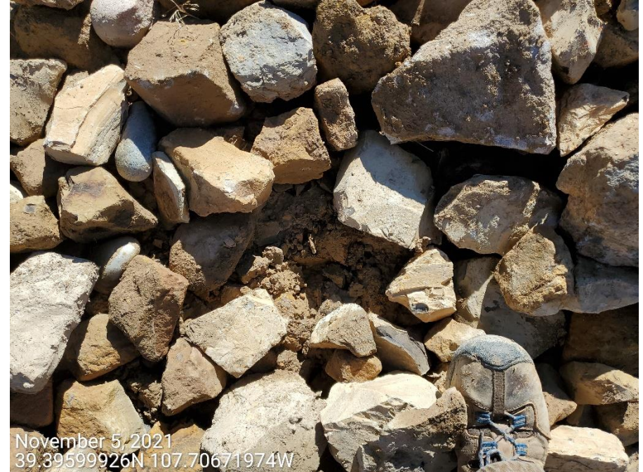
Photo 4: Photos shows the outlet from the production area leading into the sediment trap is improperly armored and missing geotextile lining per good engineering practices.
