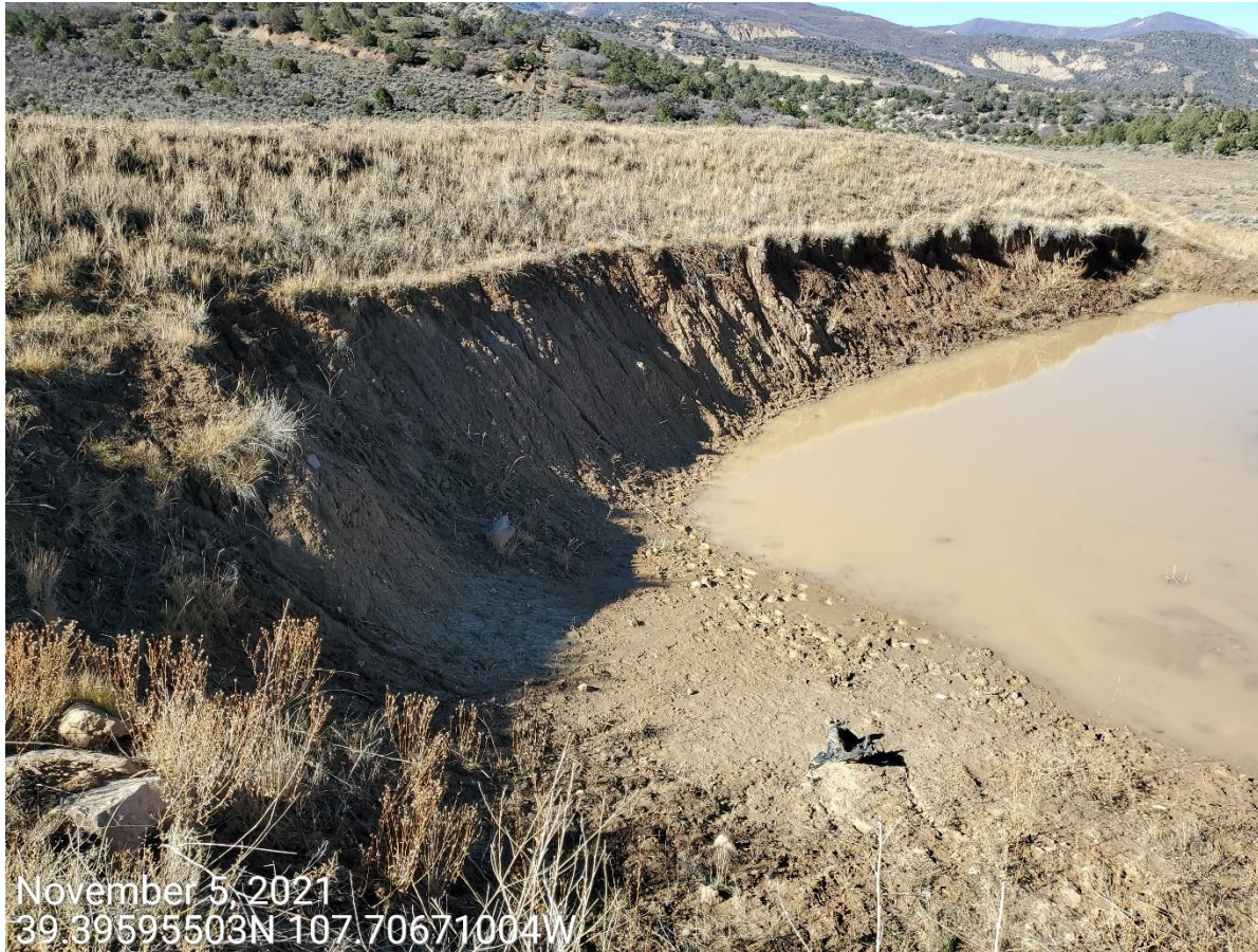
Photo 5: Photo example showing trap has been constructed with steep slopes; rill erosion evident; control measures to stabilize/protect slopes remain missing or insufficient.
