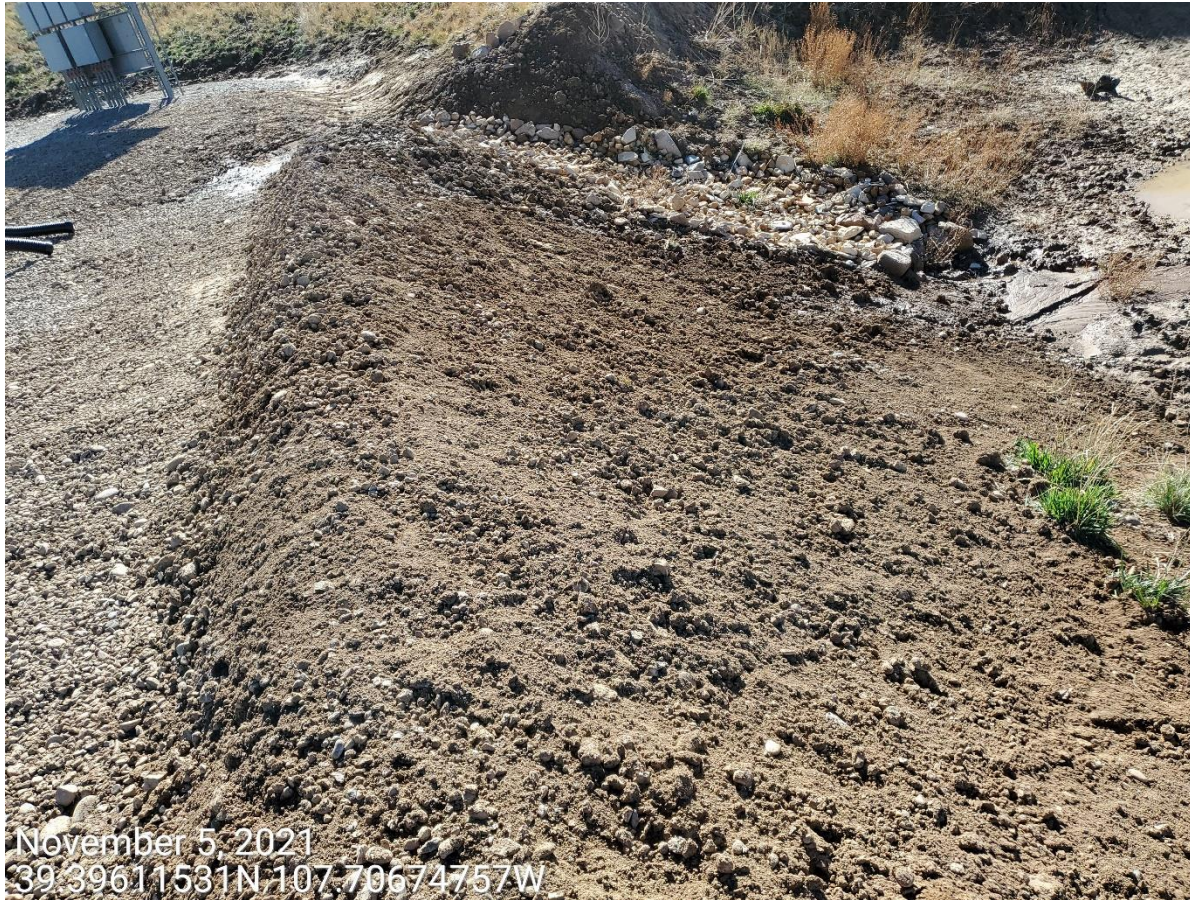
Photo 3: Continued from photo 2. Photo shows Operator has repaired erosion on the east end of the trap, however soils have been left unconsolidated; control measures to stabilize slopes of the sediment trap remain missing or insufficient.
