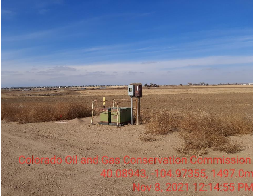
Photo 3 Unused equipment electric panel. NO METER PU us operated by gas powered motor.
