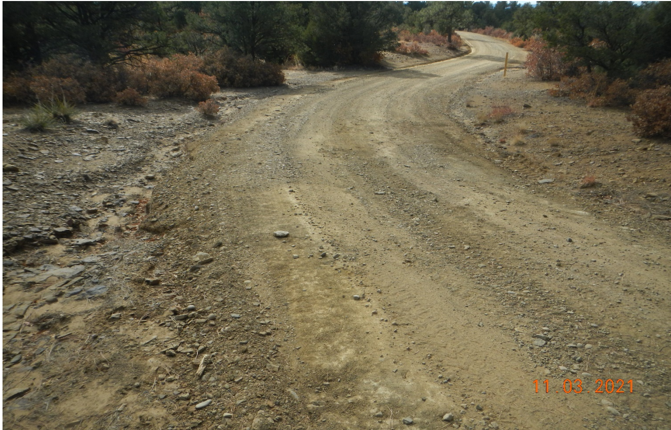
Photo 6. Facing south along the access road. The road was graded however there is insufficient stabilization.
