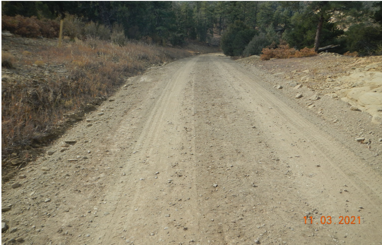
Photo 8. Facing southwest at steep road traveling down from the top of the ridge. The road was graded however loose soils are susceptible to erosion.
