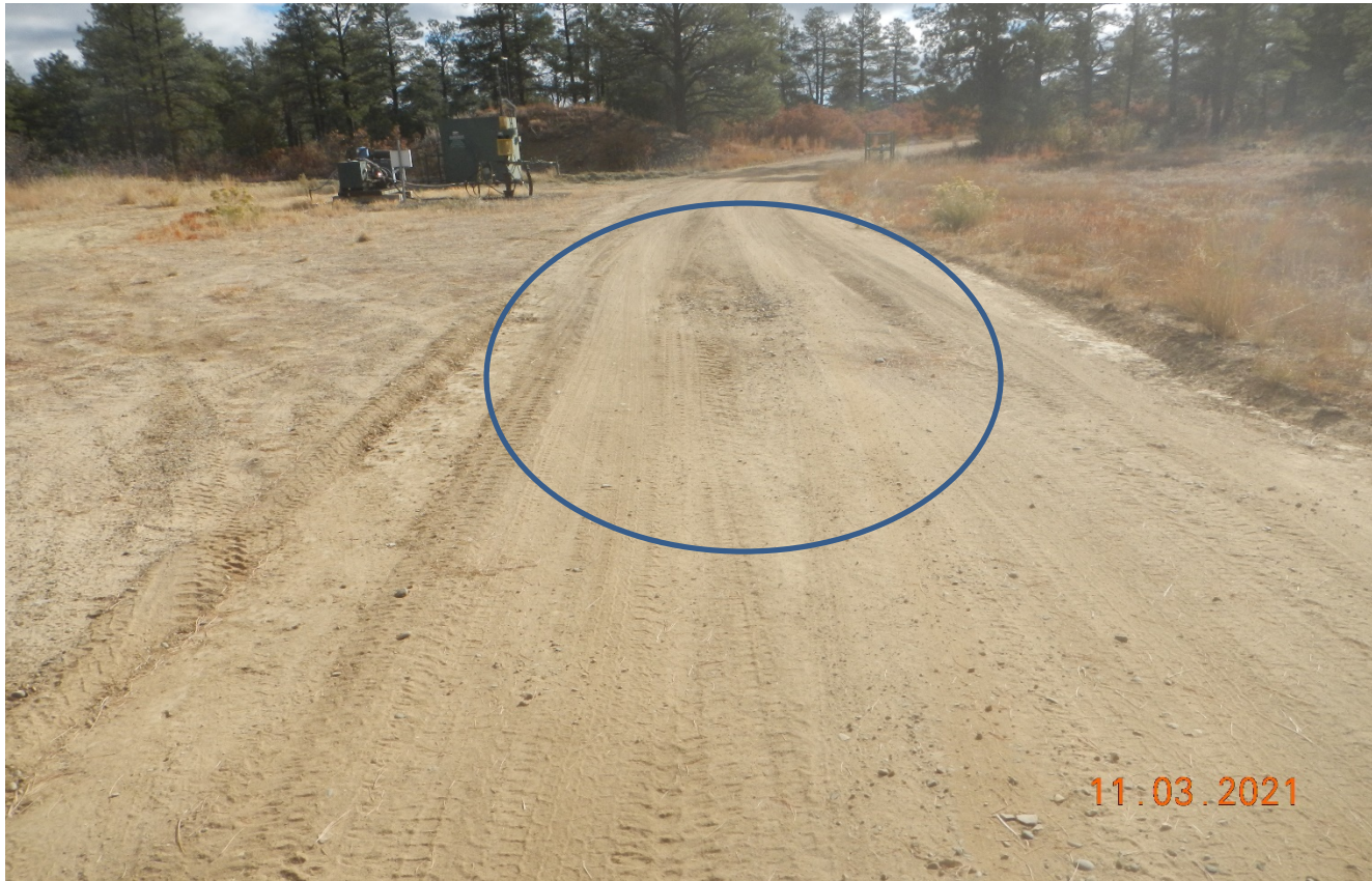
Photo 1. Facing southeast toward at the LEFT FIELD #31-29 well site. The access road was bladed however the area of water pooling circled has not been repaired to divert water. This area of the road should be crowned to divert water from the road.
