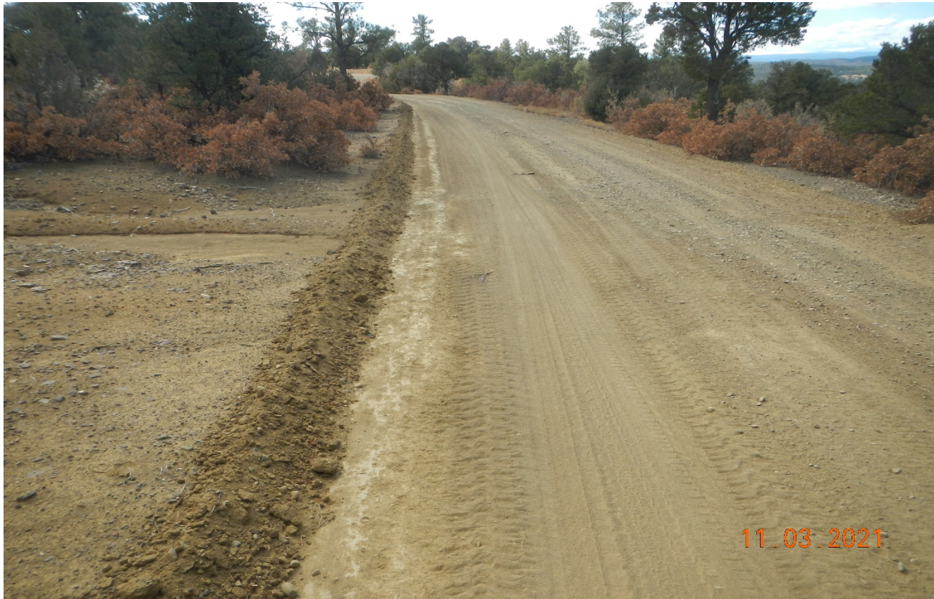
Photo 7. Facing south along the access road. The road was graded however there is insufficient stabilization. Loose graded soils are susceptible to erosion.
