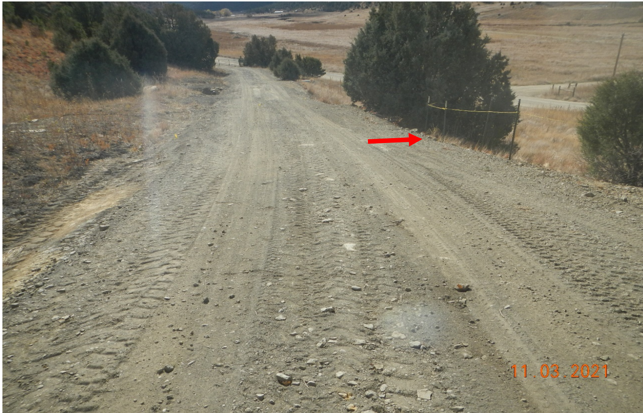
Photo 10. Facing south down the access road near county road 51. Red arrow points to where vehicle had driven off the designated road. This area down to the gate has not been restricted to prevent access by fence installation per landowner request.
