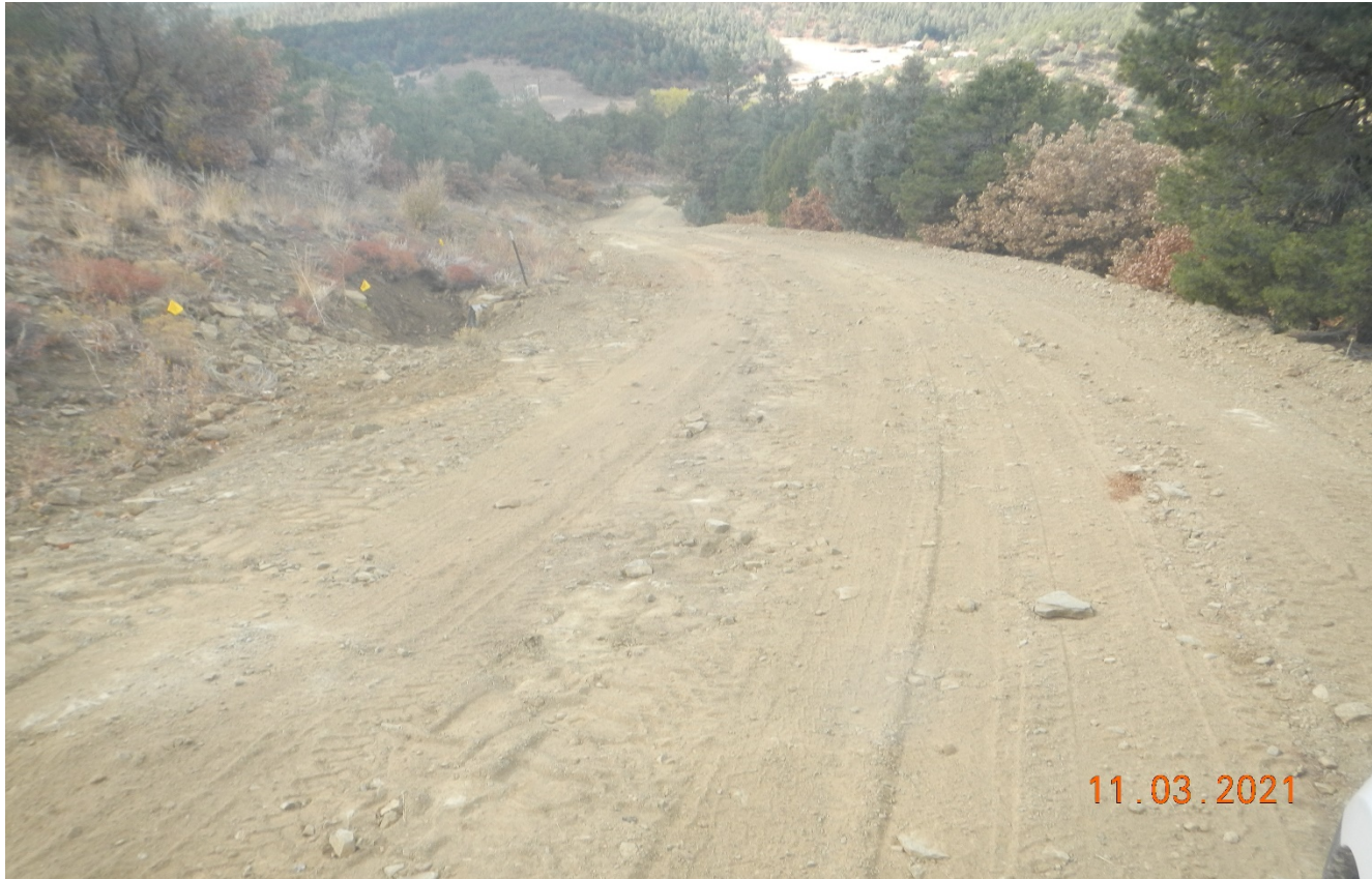
Photo 9. Facing southwest further down the hill side. The road was graded however loose soils are susceptible to erosion.
