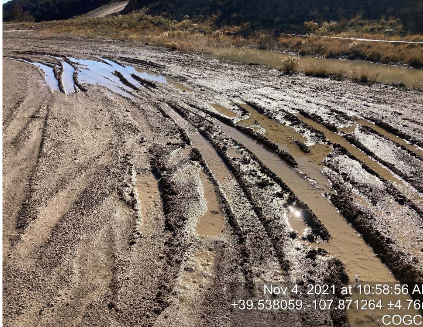
Lack of stabilization/compaction
