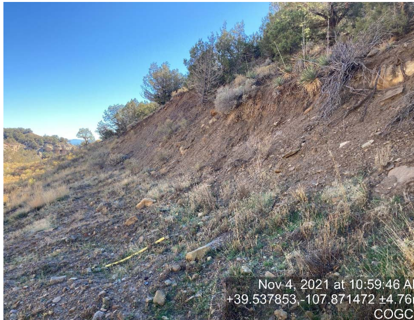
Follow up photo of erosion on cut slopes
