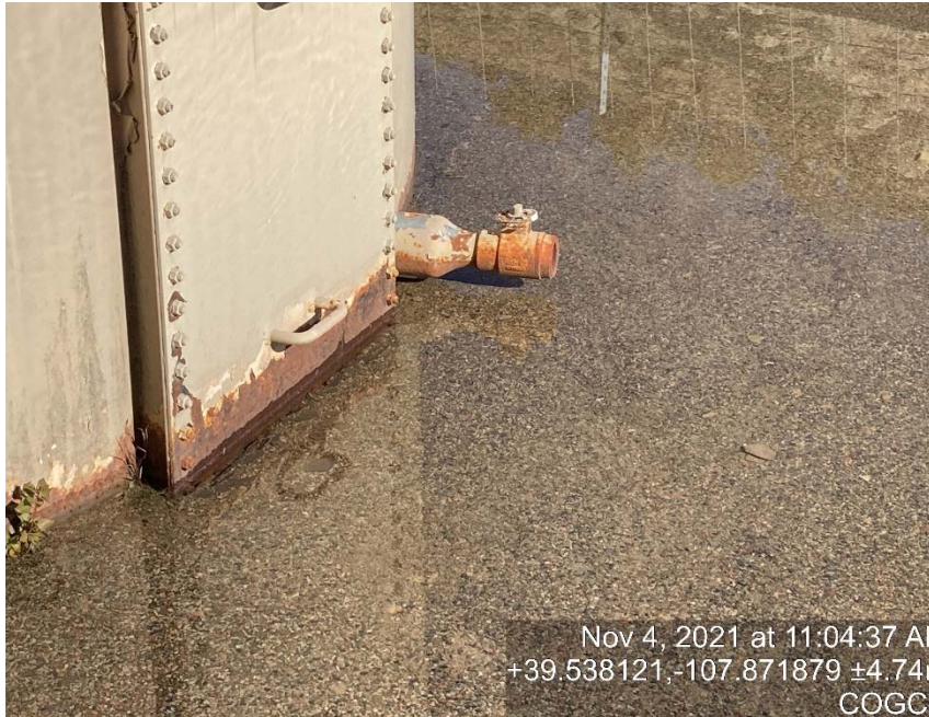
Load out line missing cap/bull plug
