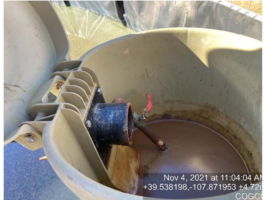
Load out line missing cap/bull plug
