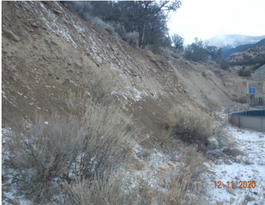
Previous inspection photo of erosion on cut slopes
