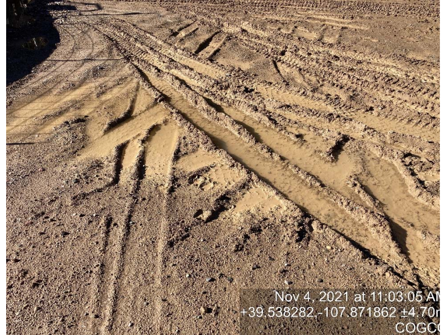
Lack of stabilization/compaction
