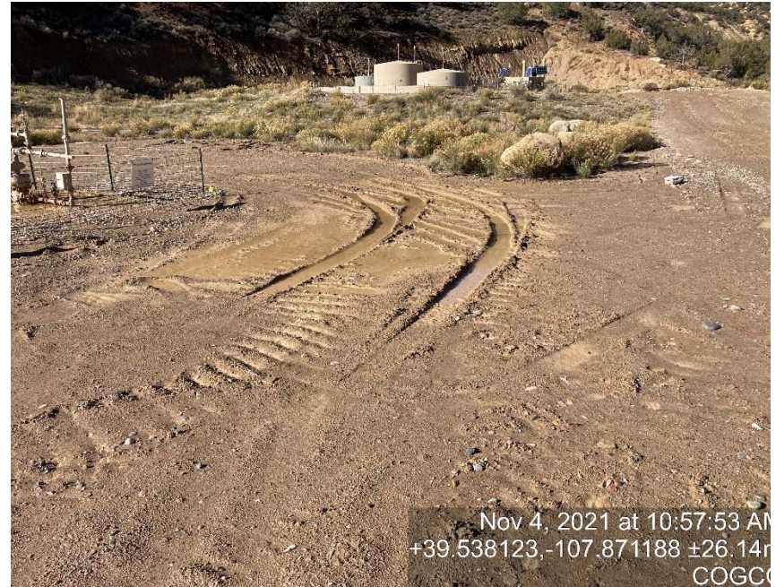
Lack of stabilization/compaction
