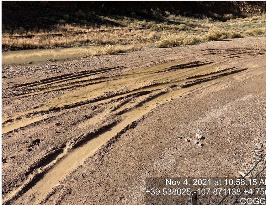
Lack of stabilization/compaction
