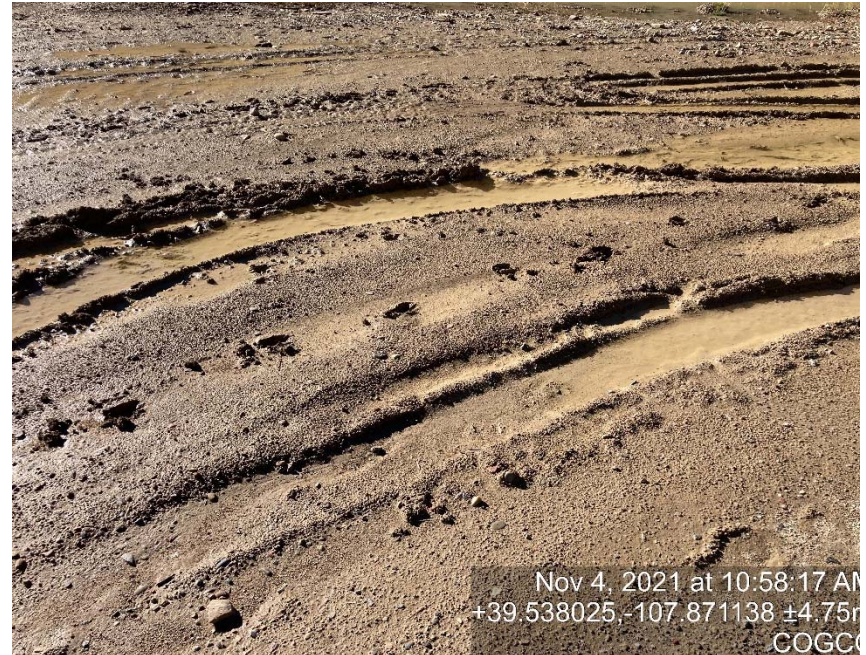
Lack of stabilization/compaction
