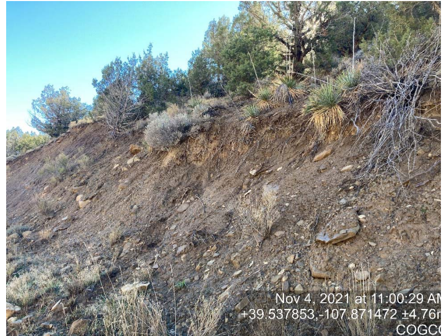
Follow up photo of erosion on cut slopes
