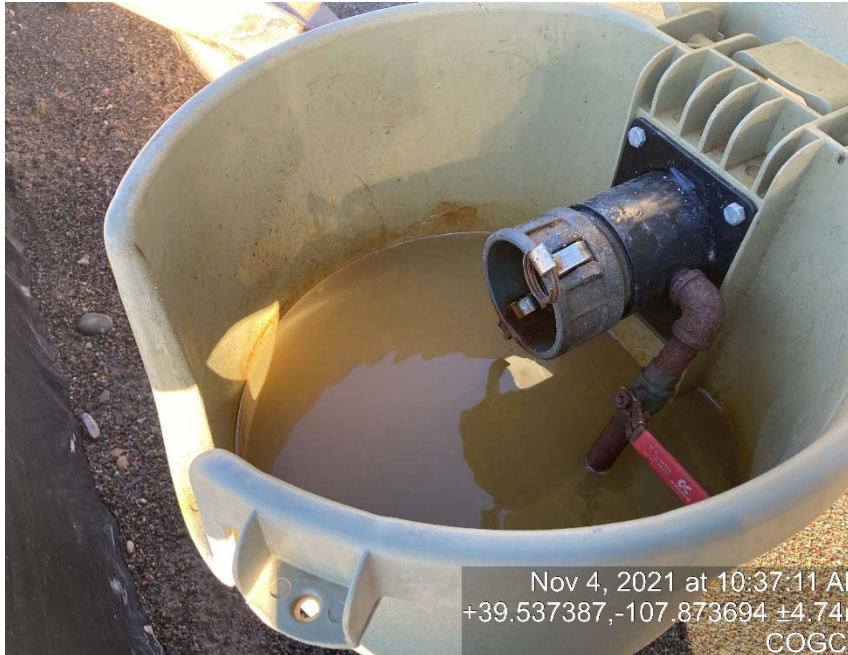
Load out line missing cap/bull plug
