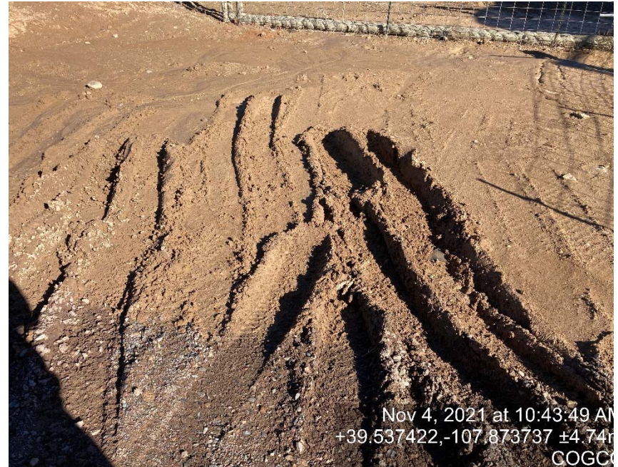
Lack of stabilization/compaction
