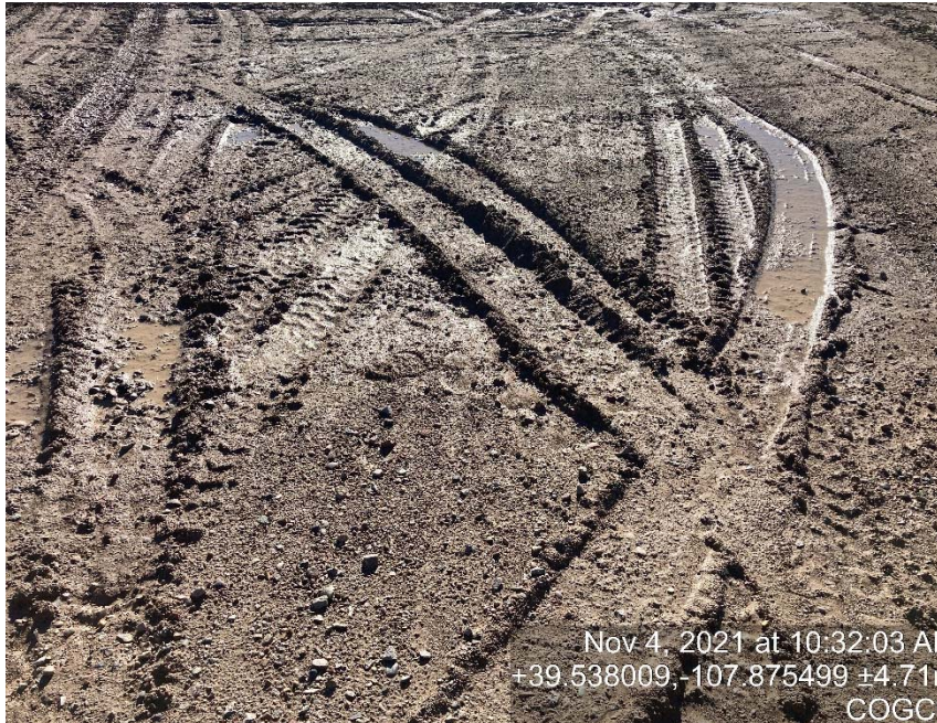
Lack of stabilization/compaction
