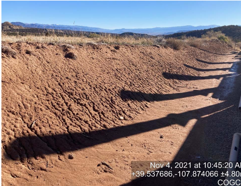
Lack of stabilization/erosion
