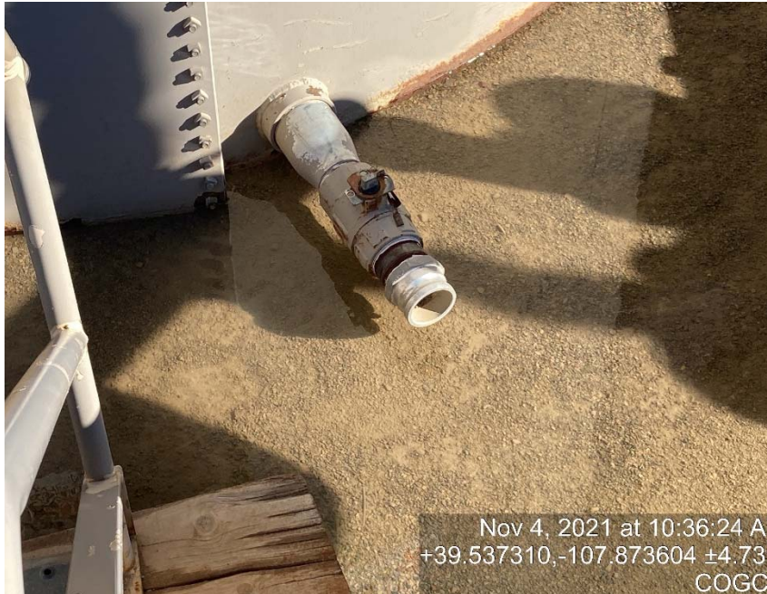
Load out line missing cap/bull plug
