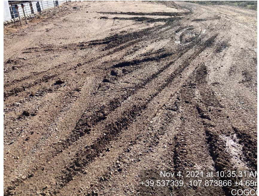
Lack of stabilization/compaction
