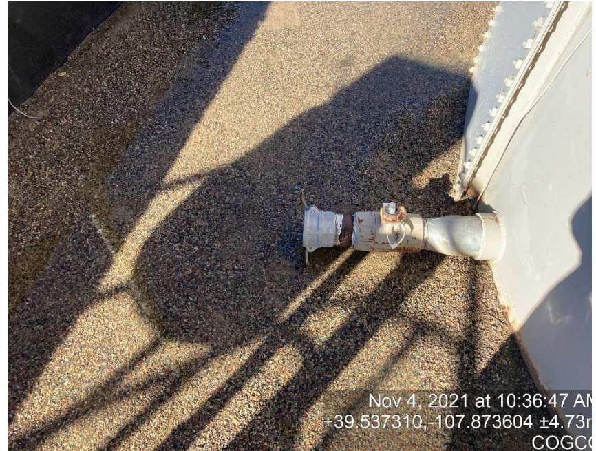
Load out line missing cap/bull plug
