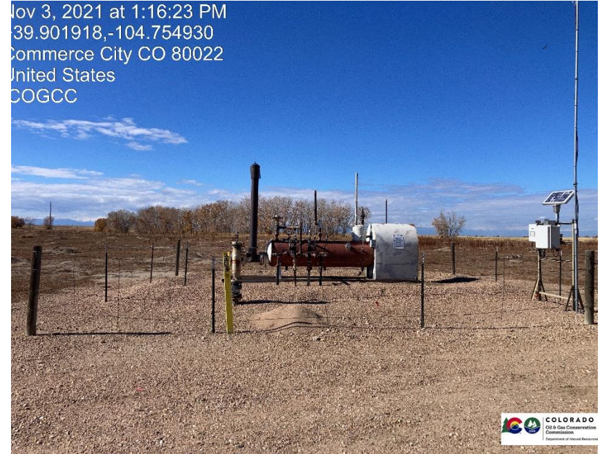
Pic 2 Separator, automation equipment.
