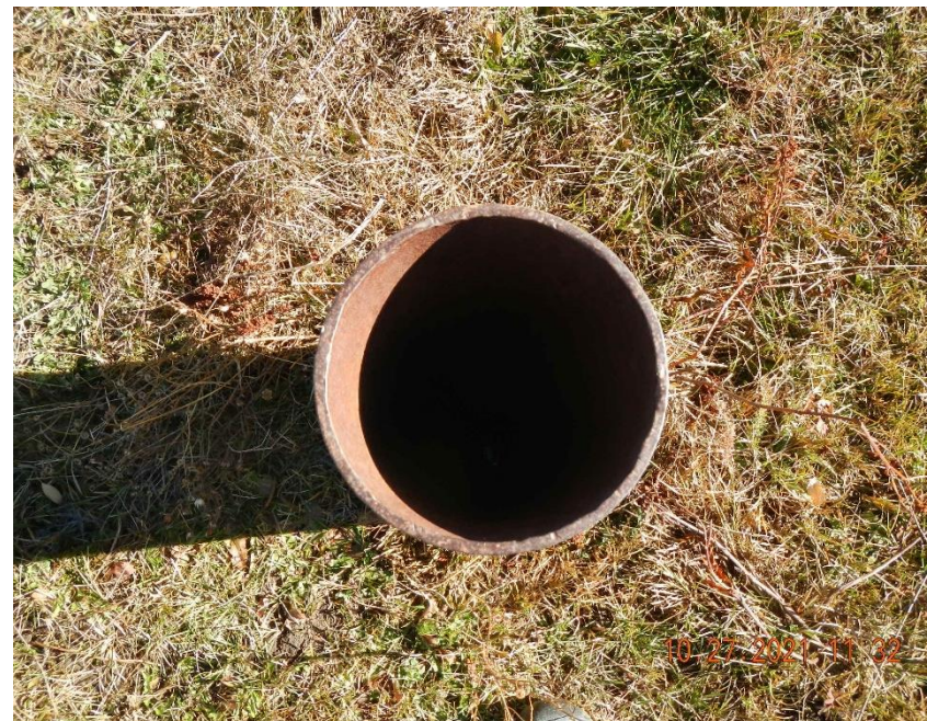
Underwood Ditch (OWP) #4 casing. Water was visible within casing during this inspection.
