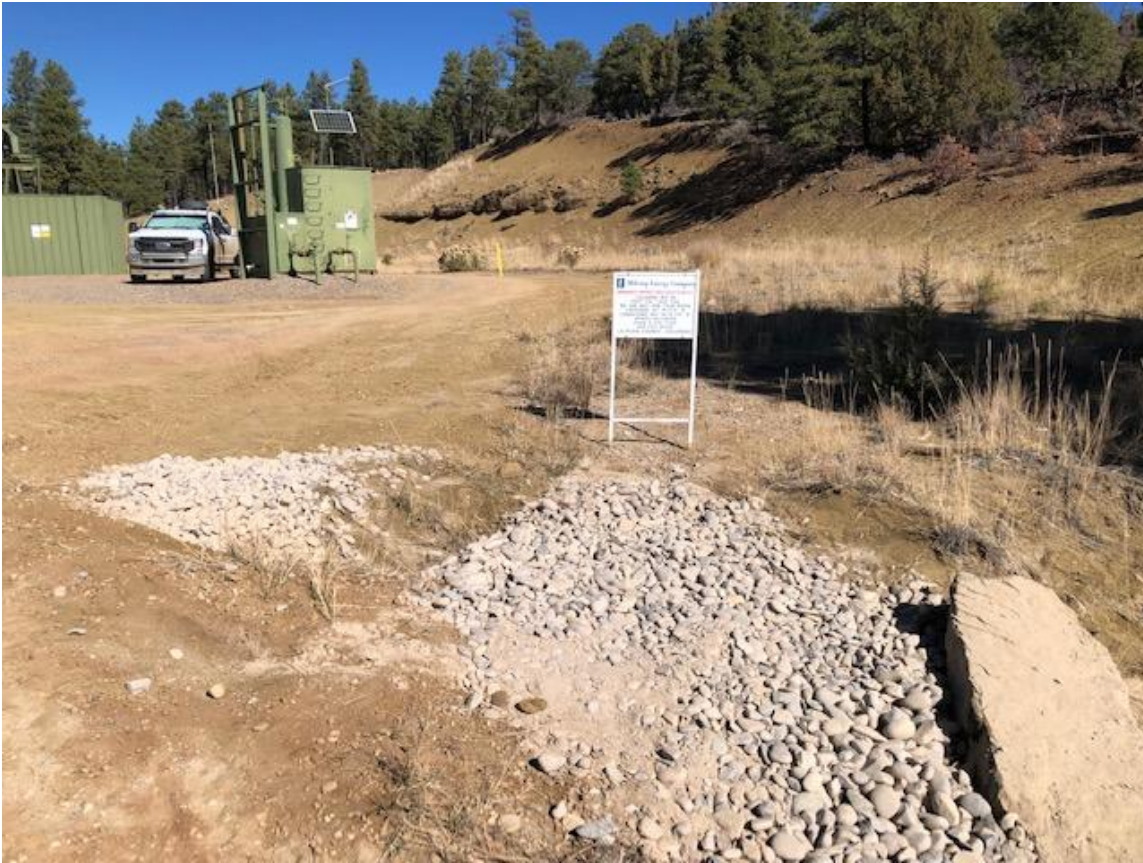
Storm Water stabilization installed.
