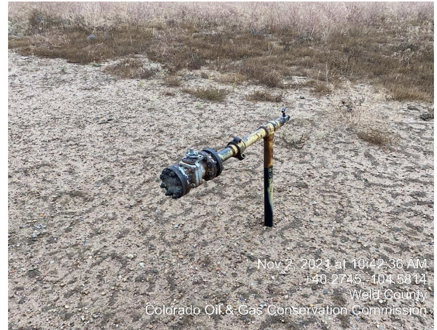
Photo #5 Unmarked Riser
