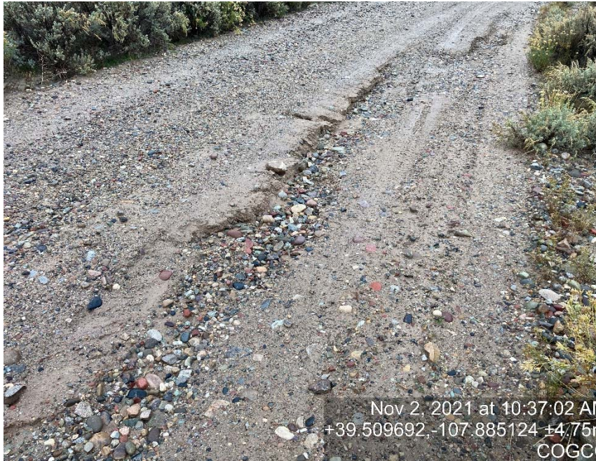
Erosion on access road
