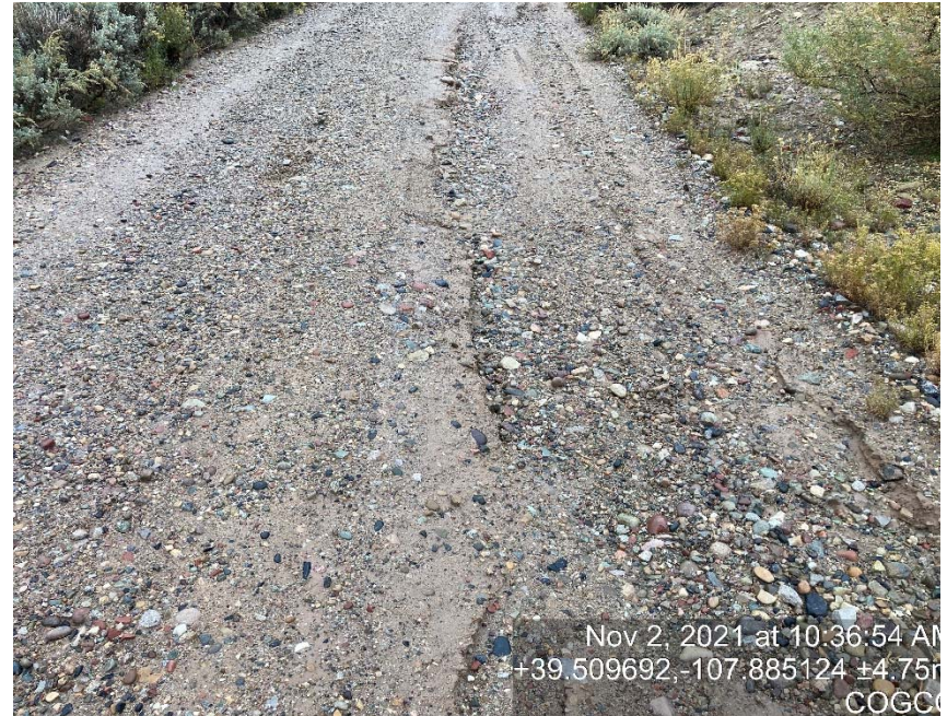
Erosion on access road
