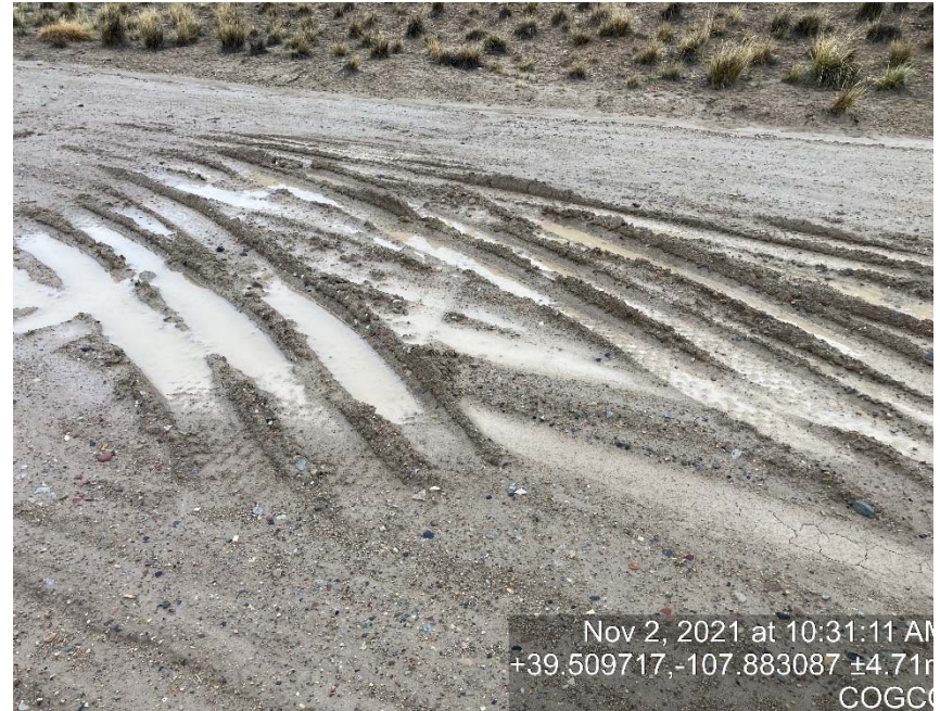
Lack of stabilization/compaction
