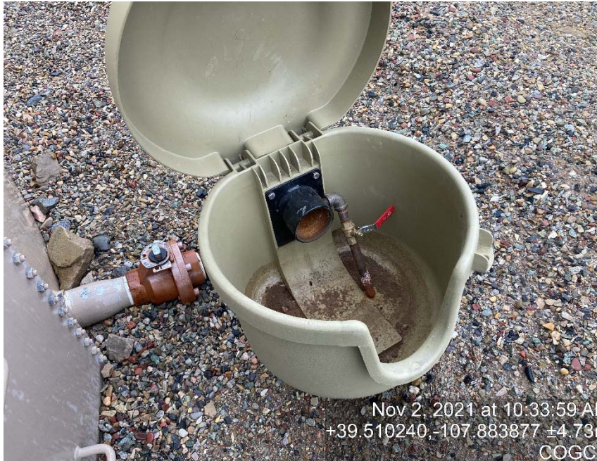
Load out line missing cap/bull plug
