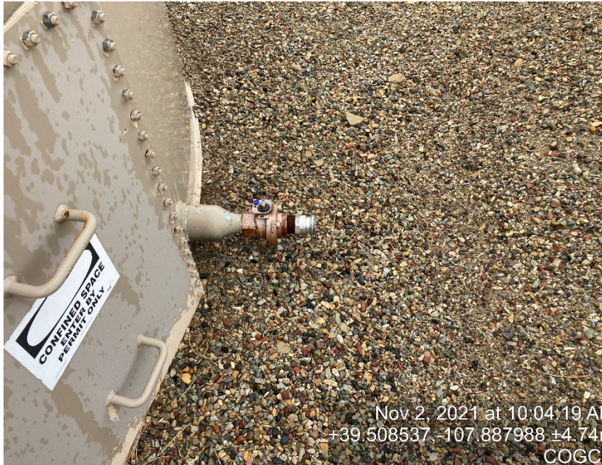
Load out line missing cap/bull plug
