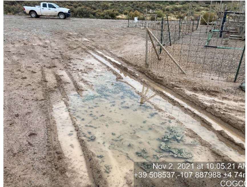
Lack of stabilization/compaction
