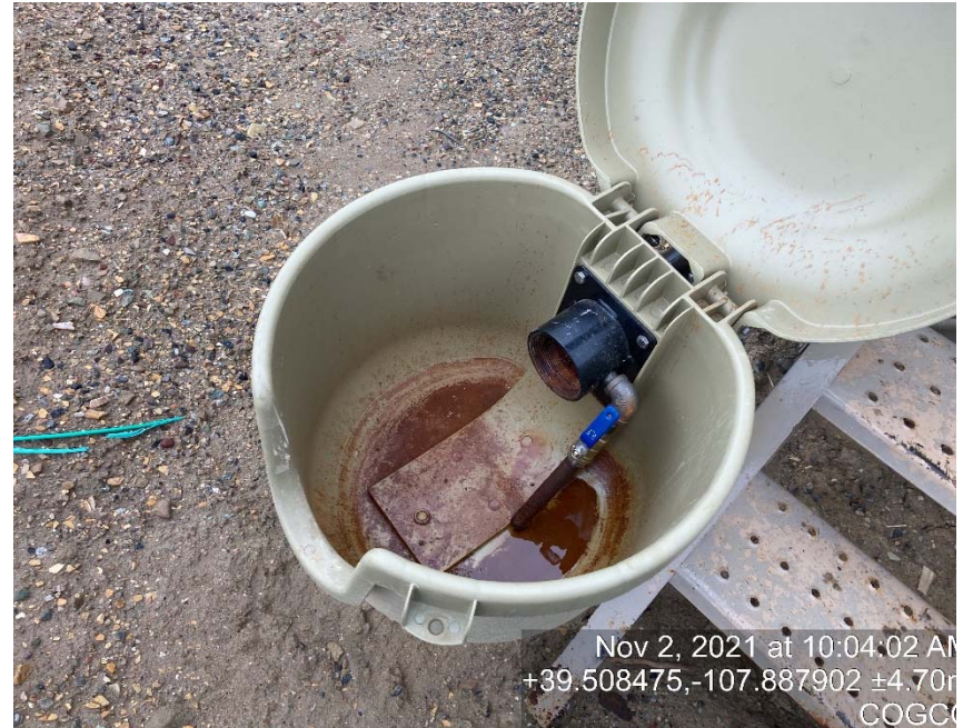
Load out line missing cap/bull plug
