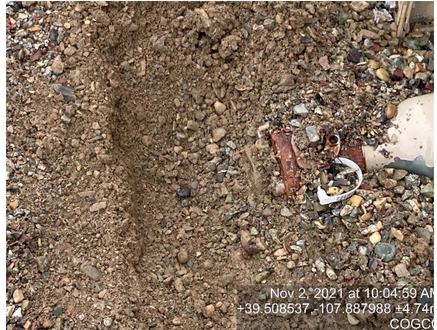
Load out line missing cap/bull plug
