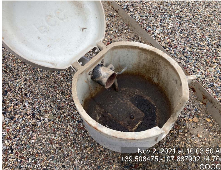
Load out line missing cap/bull plug
