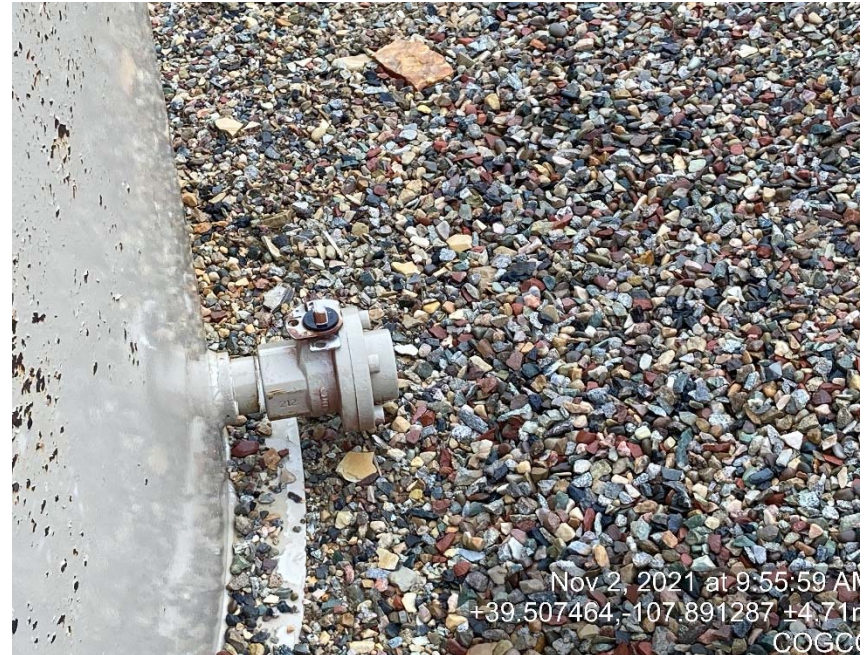
Load out line missing cap/bull plug
