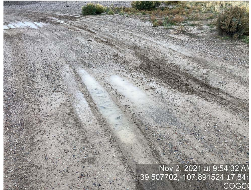
Lack of stabilization/compaction
