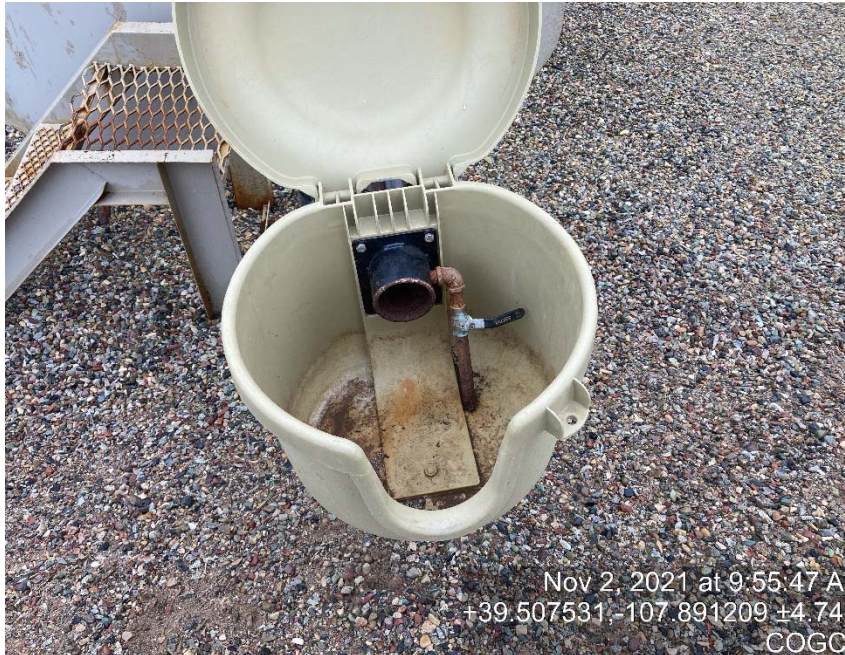
Load out line missing cap/bull plug
