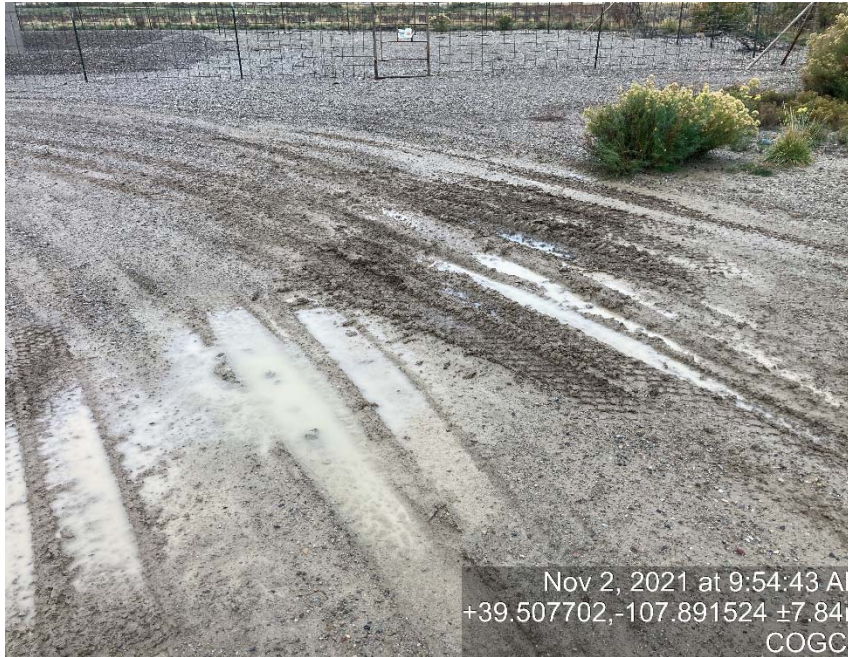
Lack of stabilization/compaction
