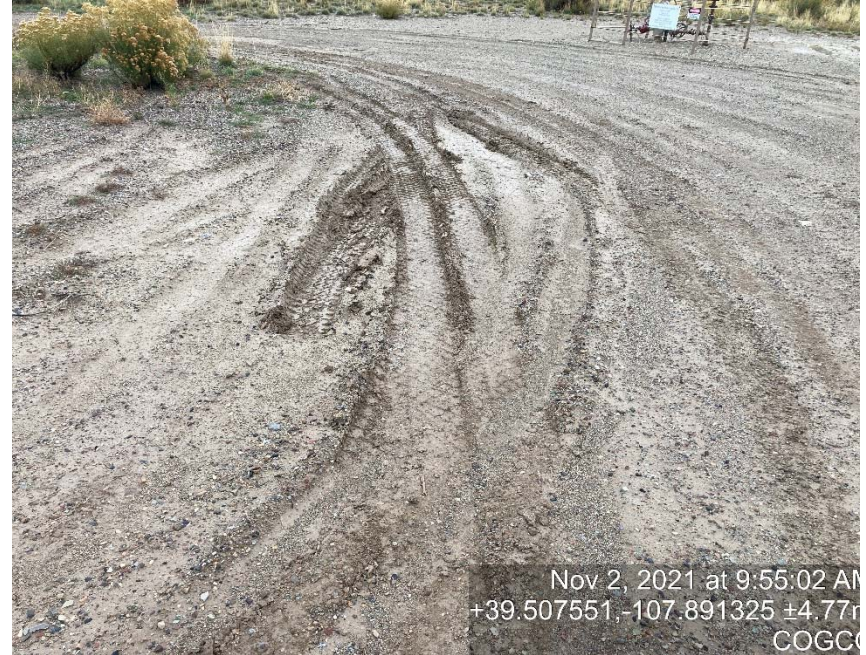
Lack of stabilization/compaction
