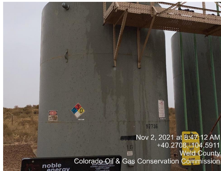
Photo #3 Missing Capacity Label
