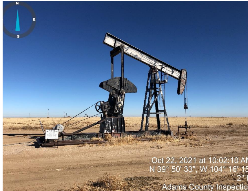
Photo #1 Pump Jack.
