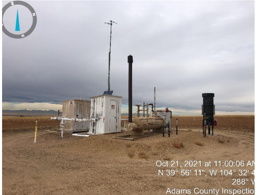
Photo #2 Meter run, ECD & separator.
