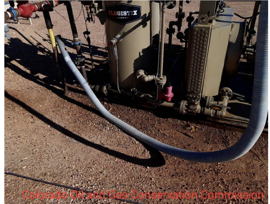
Photo 6 Stained soil around compressor skid.
