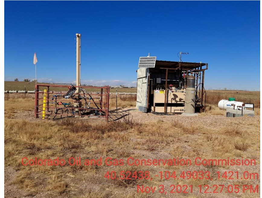
Photo 2 Well head and HYD motor skid
