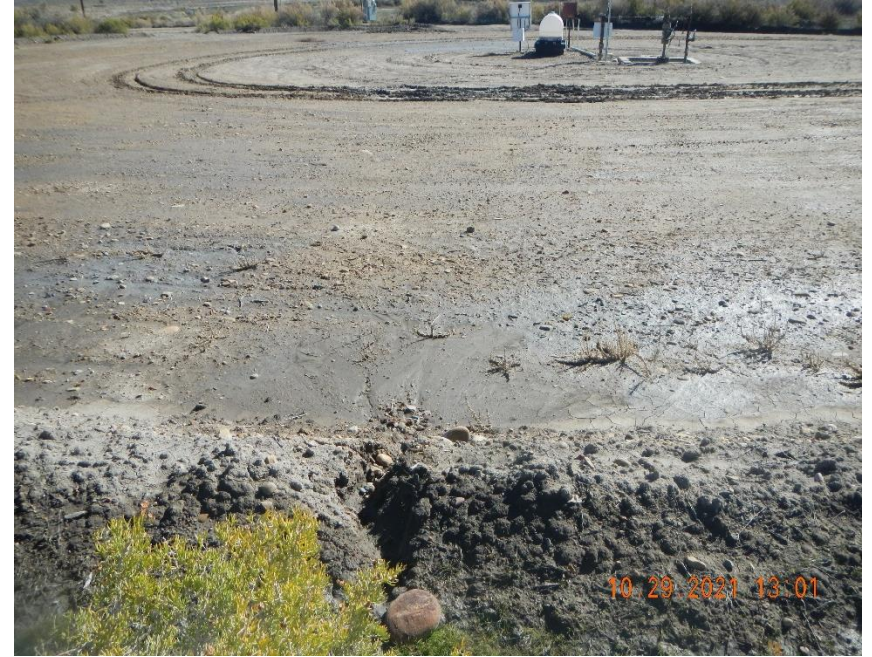
Erosion rill breaching berm wall.
