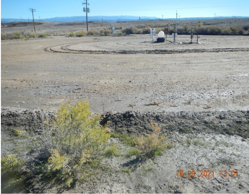
Erosion rill breaching berm wall.
