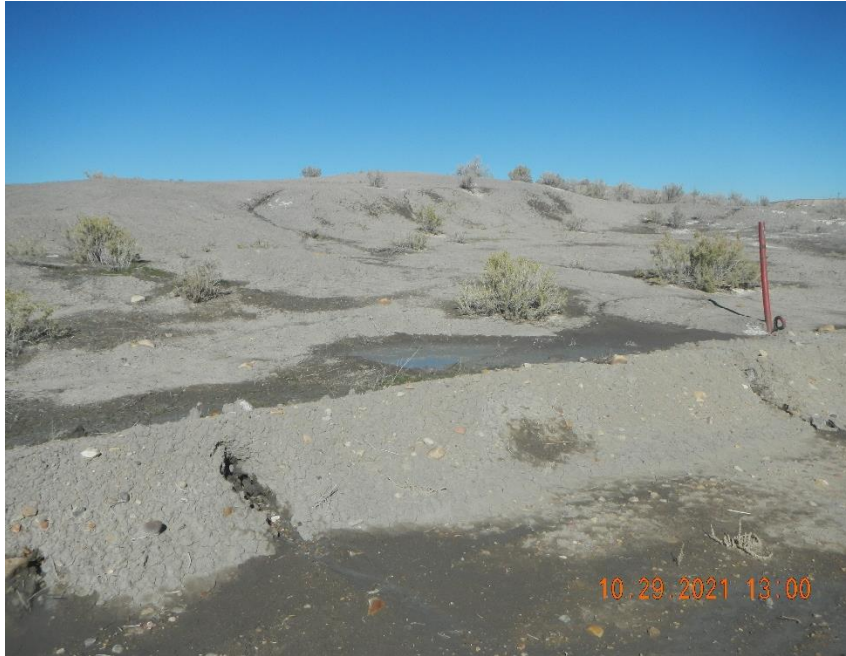
Erosion rill breaching berm wall.
