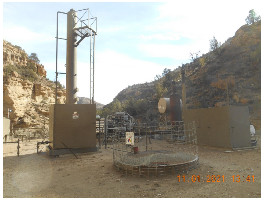
Dehydrator, Separator and blowdown tank
