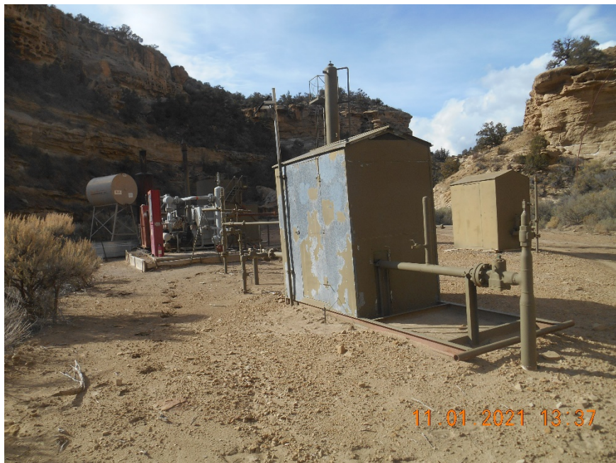
Compressor and Meter housings
