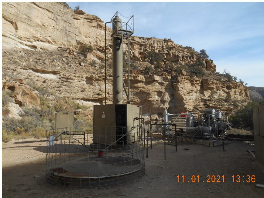
Dehydrator, blowdown tank and compressor
