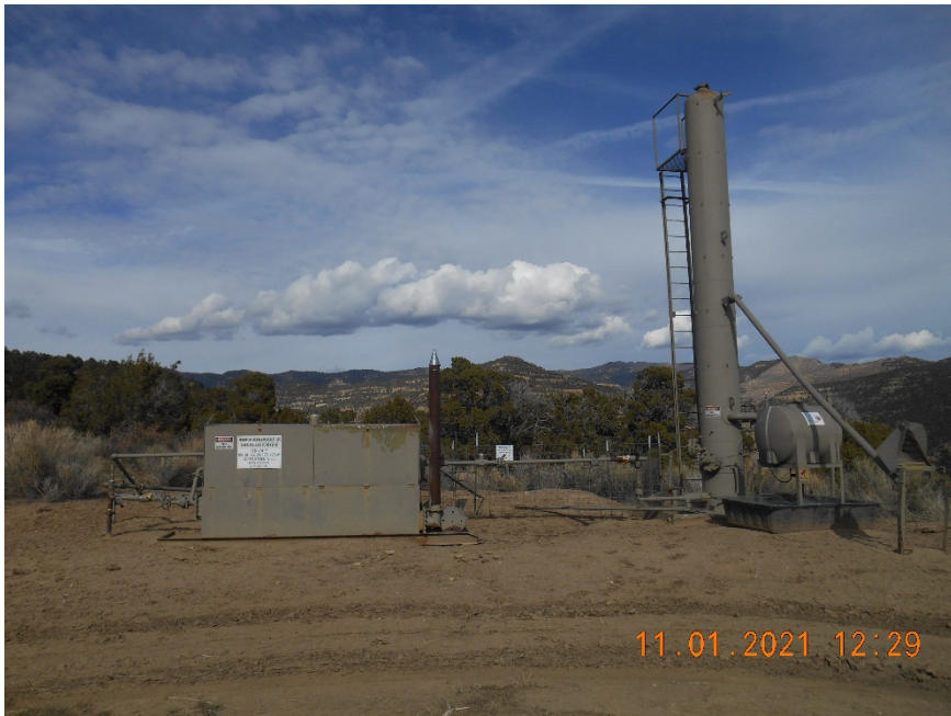
Separator and Dehydrator
