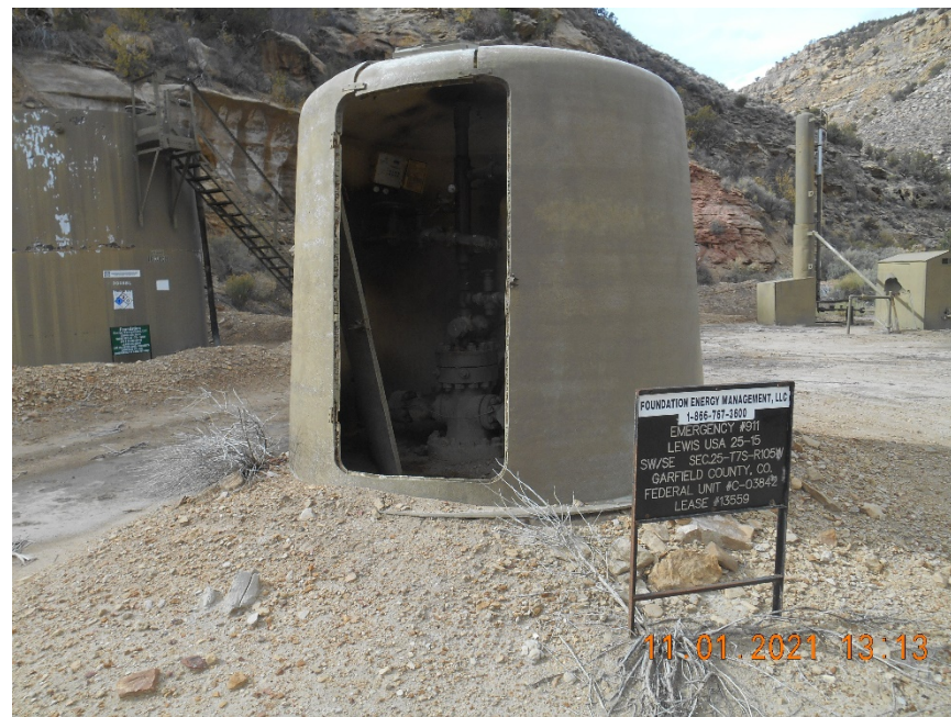
Wellhead inside housing with signs.
