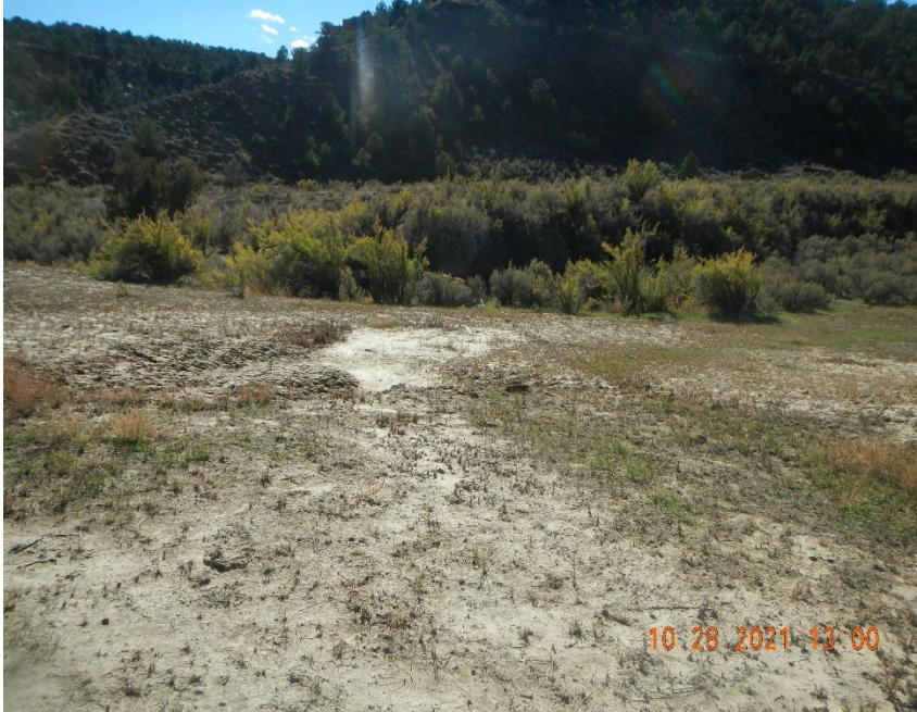
Storm water erosion and movement of sediment off south west corner of location.
