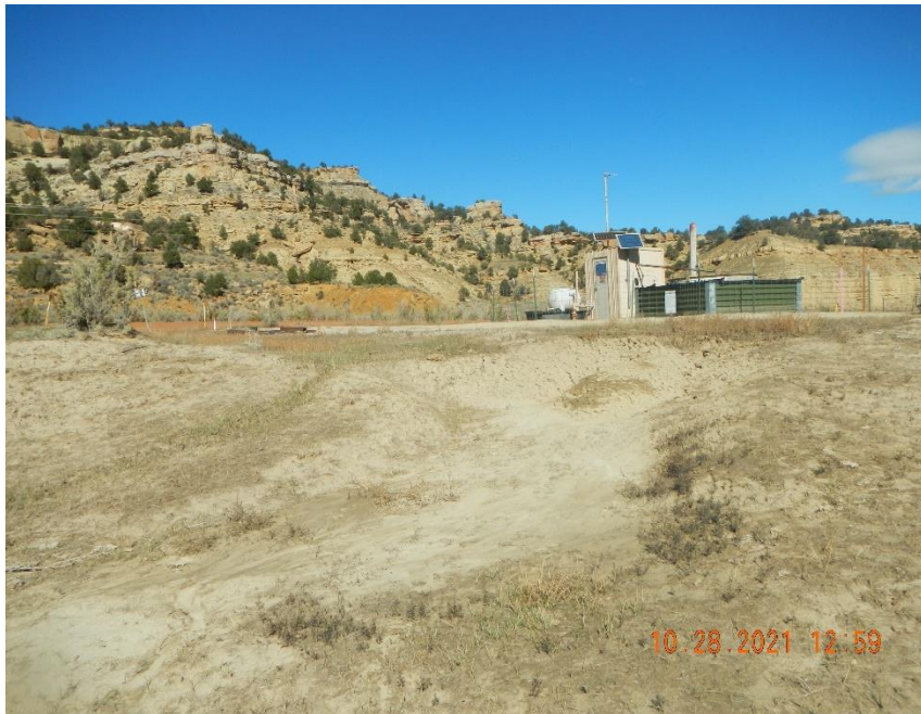
Storm water erosion and movement of sediment off south west corner of location.
