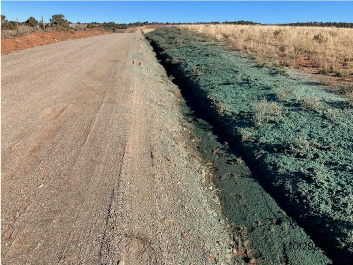
**Soil amendments were applied to the slope and the slope was seeded with a landowner-approved seed mix. The slope was then covered with hydromulch to stabilize the slope.**
