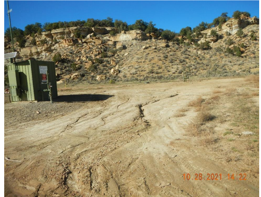
Movement of sediment. Erosion rills running on access to CR 116 ditch.
